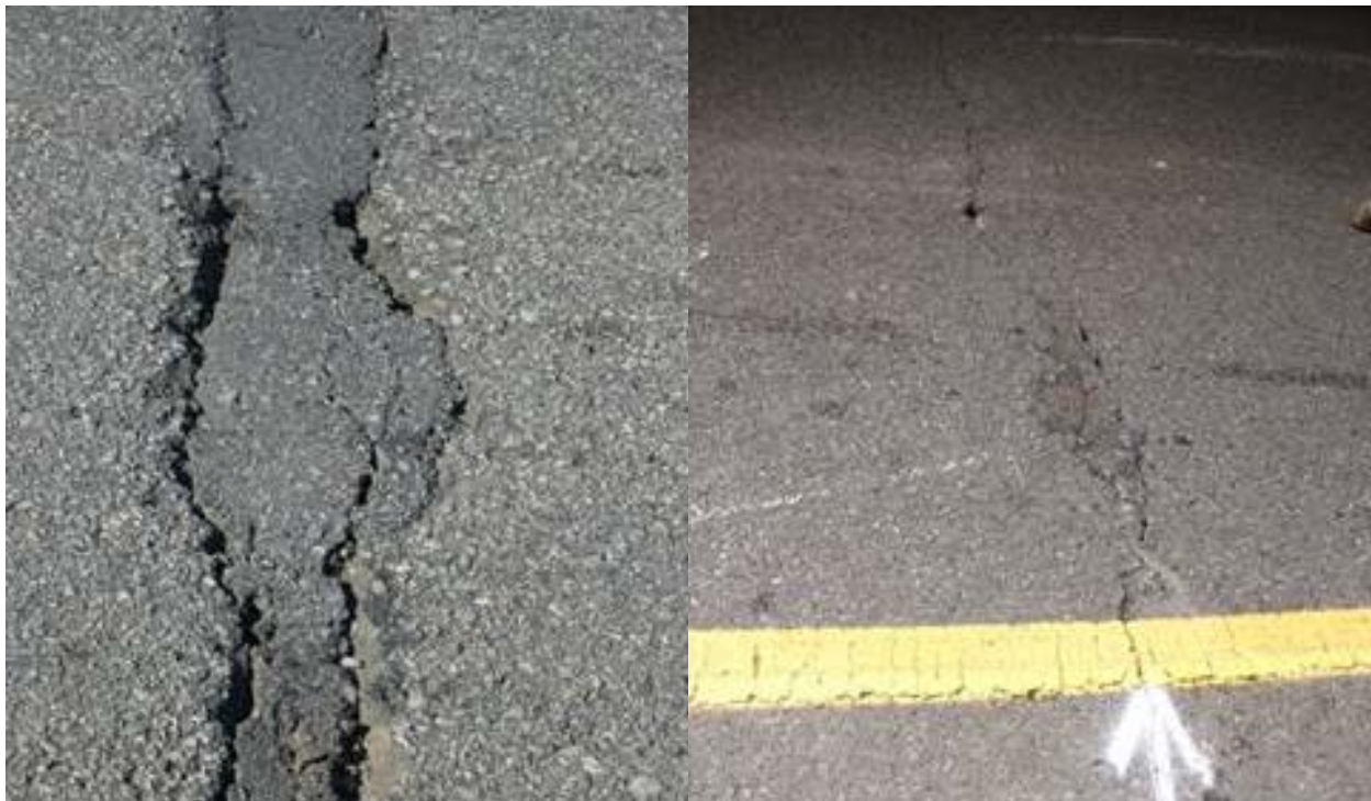
Figure 4. Illustrative Pavement Conditions Prior to Stop-Gap Overlay
