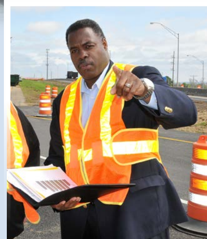
AHTD Assistant Chief Engineer for Operations Emanuel Banks stressed the need for driver safety in the Interstate 540 construction zone.
