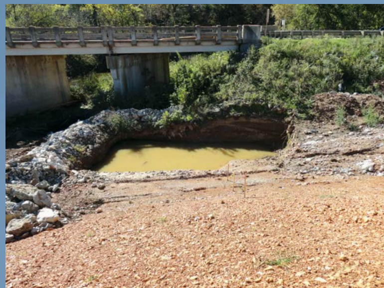
(Top and Center) Silt fence lining the water's edge to minimize sediment impacts. (Bottom) Sediment basins catch muddy water before it leaves the construction site.
