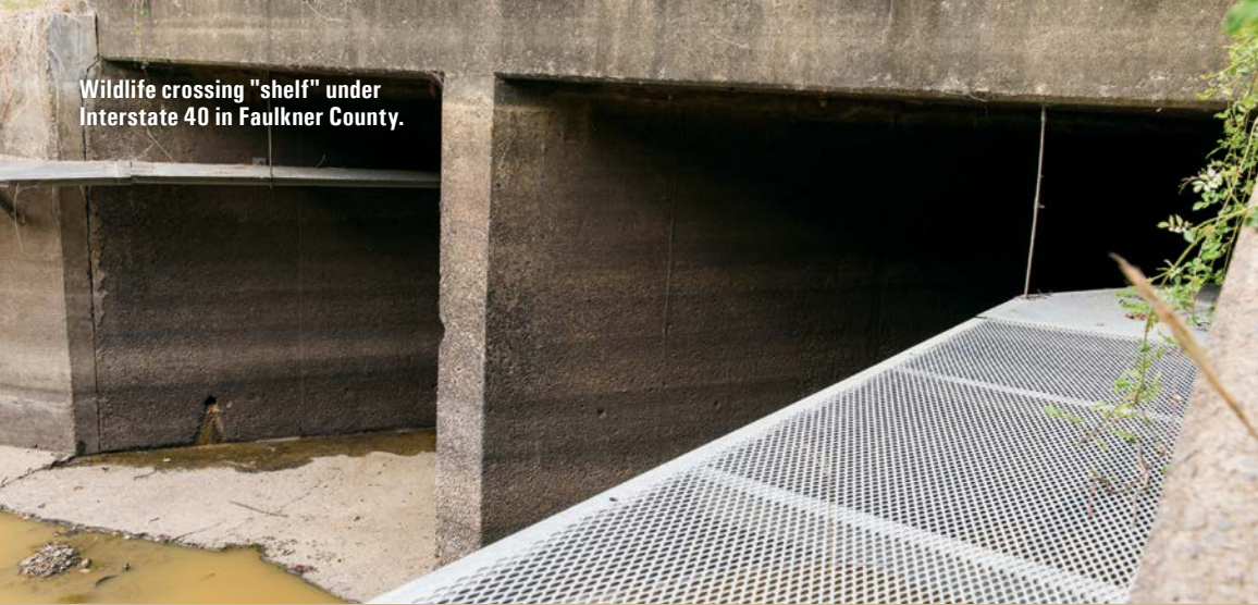
A wildlife "bench" providing safe passage under Interstate 40.
