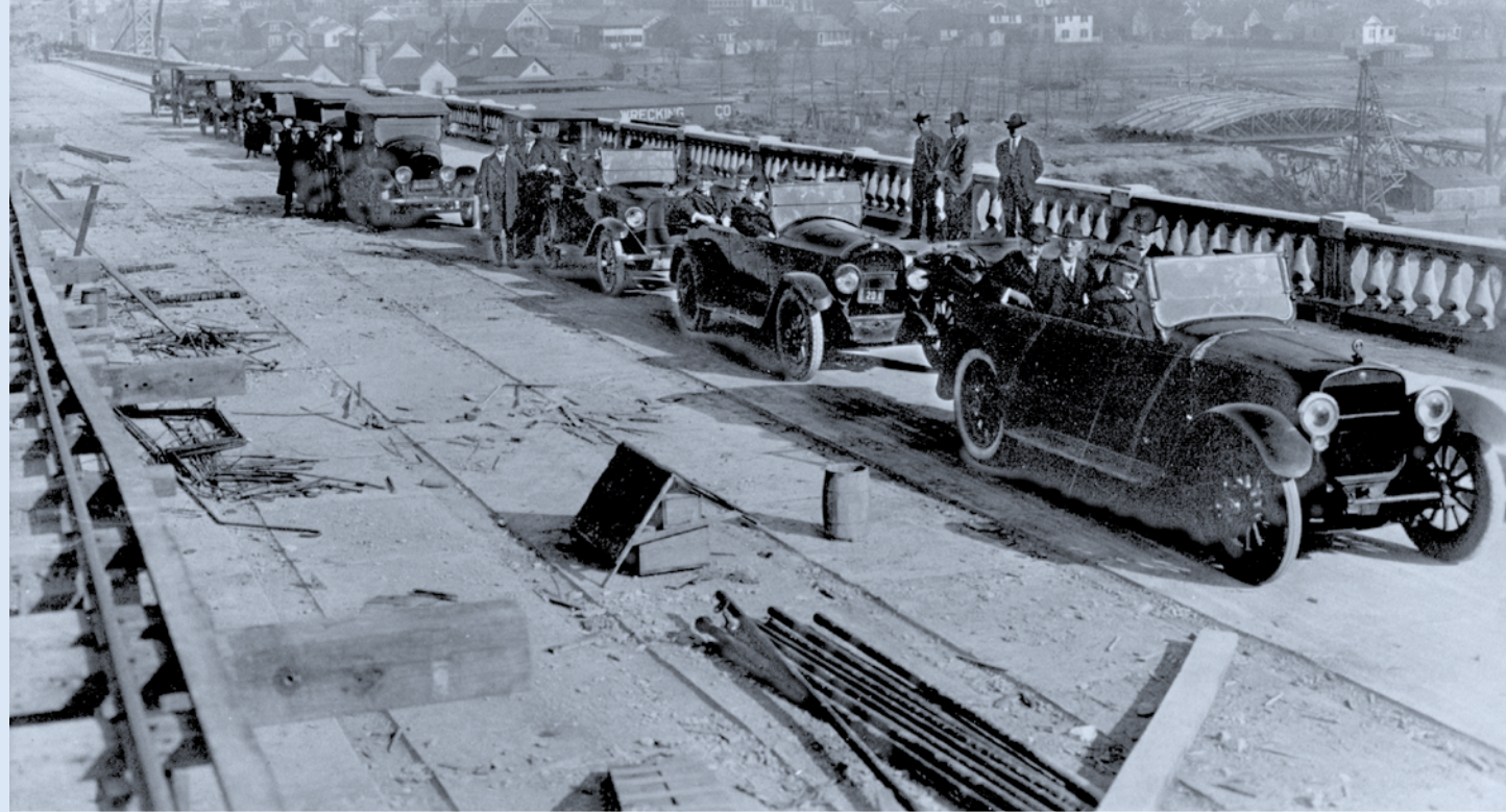
DECEMBER 25, 1922: Broadway Bridge Improvement District Commissioners were the first ones to drive over the Broadway Bridge prior to its opening.
