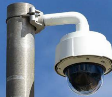
Traffic Camera on Interstate 430 at Colonel Glenn Road Exit
