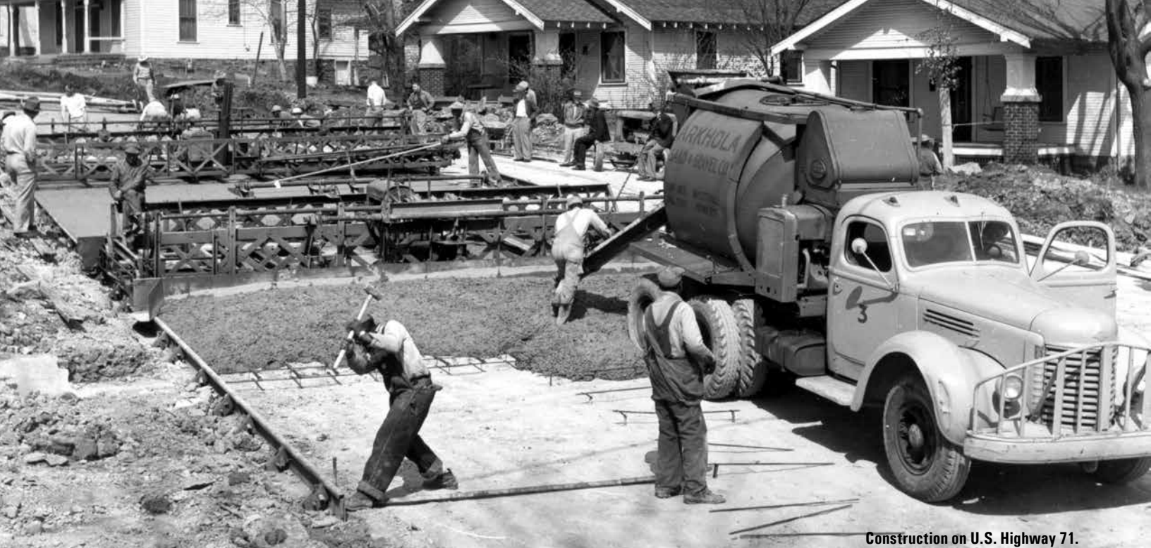
Construction on U.S. Highway 71.
