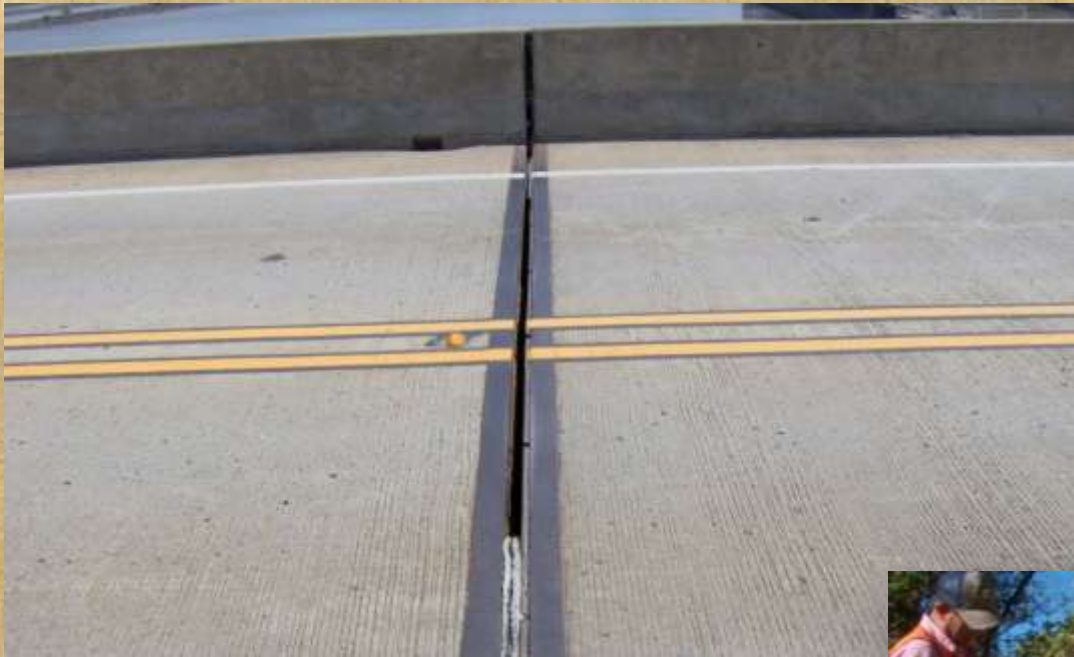
Typical Failed Bridge Joint
