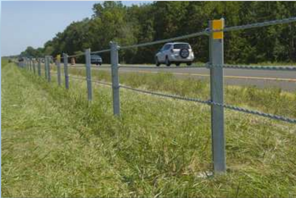
Cable Median Barrier
