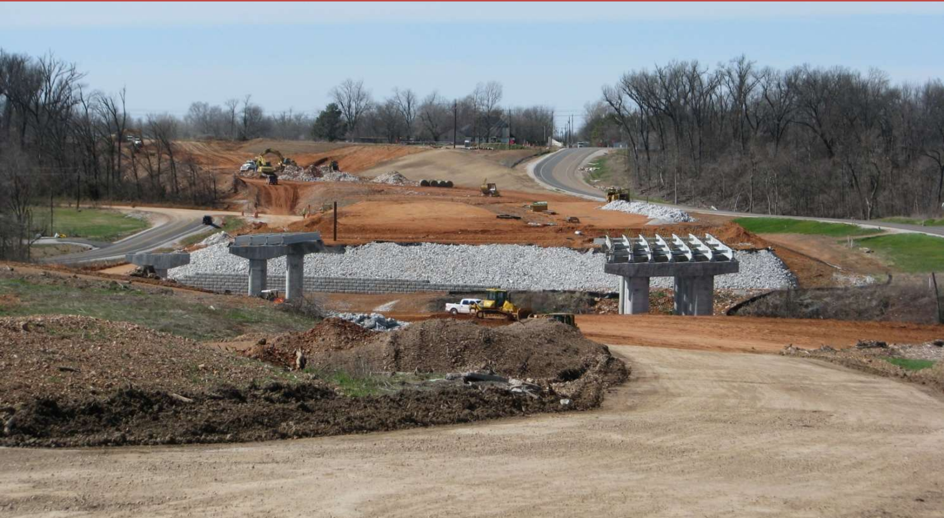
Main Lanes & Ramp EN Bridges over Puppy Creek
