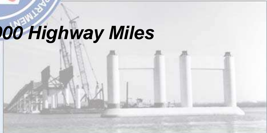
I-430 River Bridge, 1973
