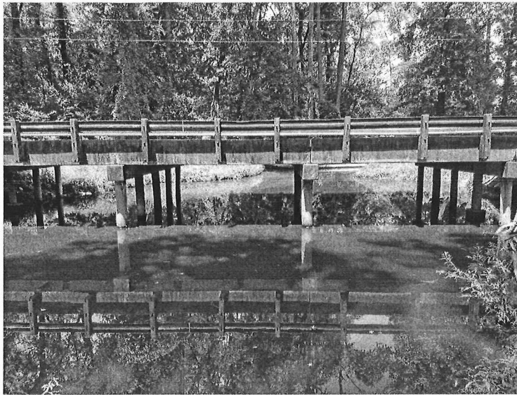
Figure 2. Bridge over Halfway Creek looking north.
