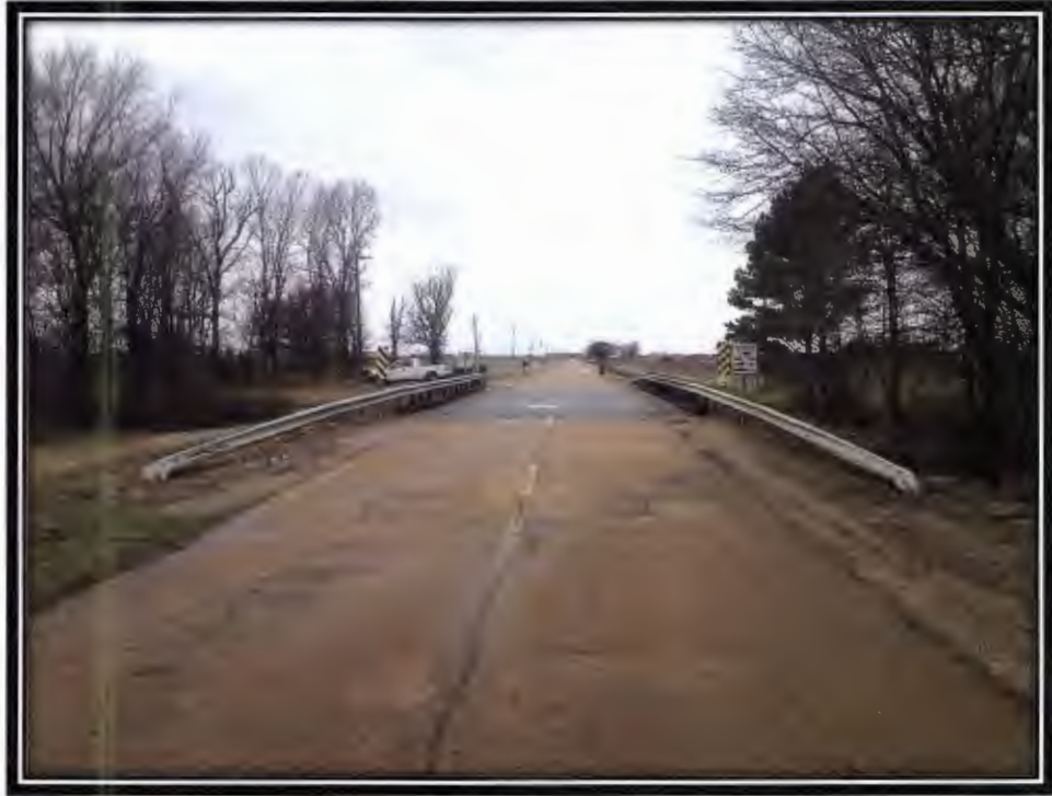
Hwy. 144 bridge over Main Ditch in Chicot County.
