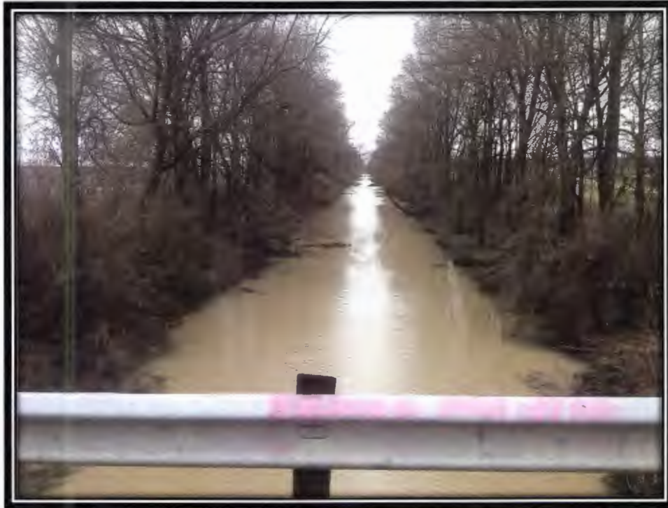
Downstream of existing bridge.
