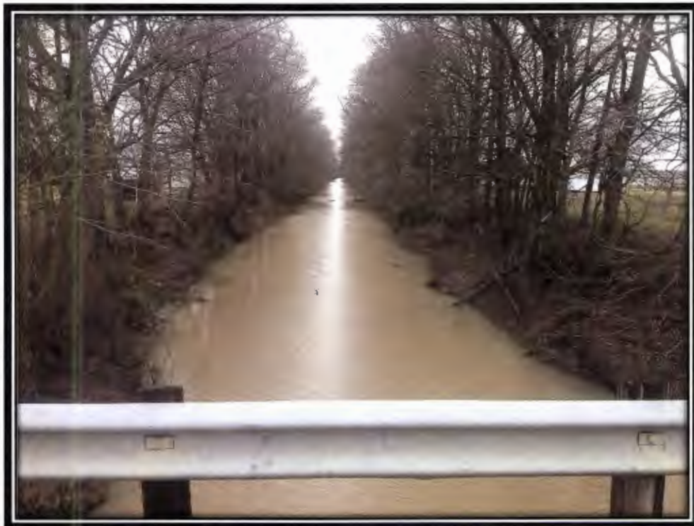
Upstream of existing structure.
