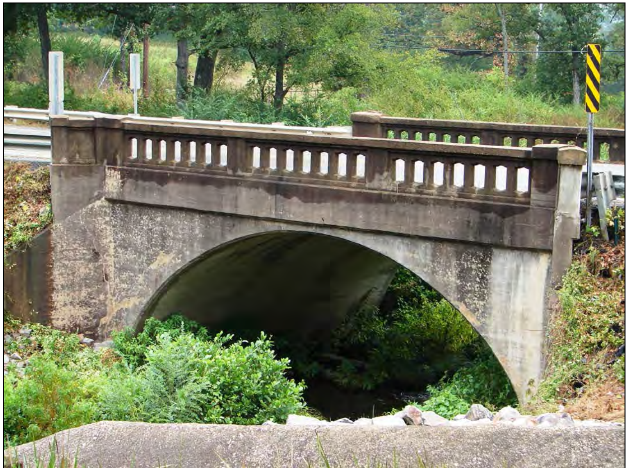
Figure 1. AHTD Bridge Number 01345
