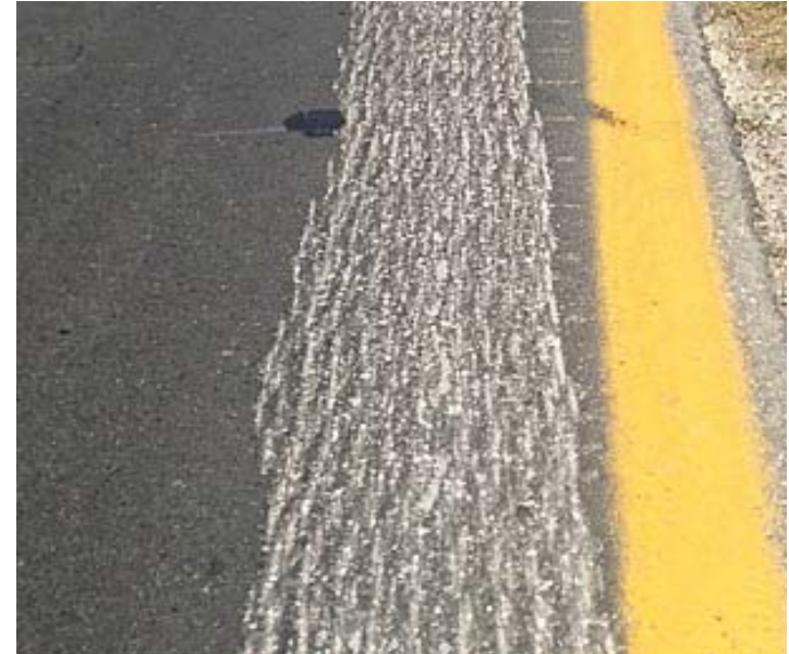
Grinding visually apparent on new asphalt pavements (waterblastingtechnologies.com)
