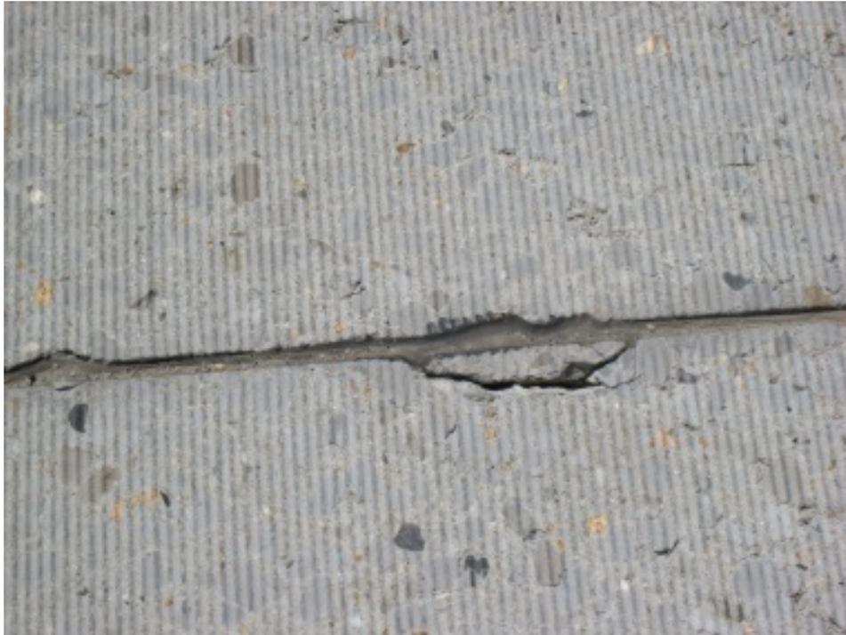
**Figure 55. Early Transverse Joint Deterioration**
