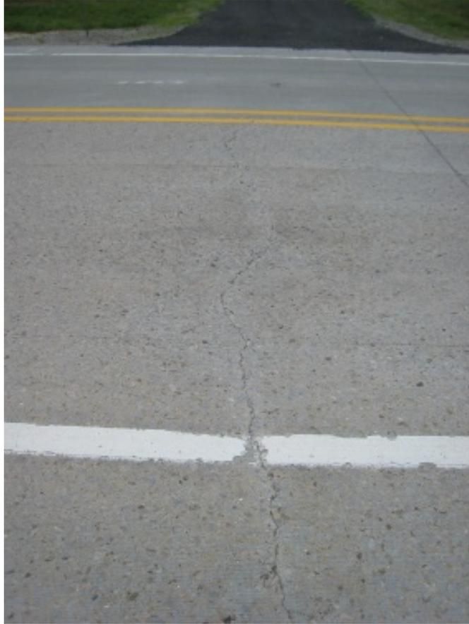
**Figure 68. Full Lane Width Crack – Station 199+90**
