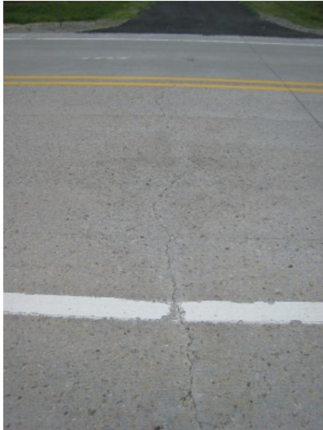
**Figure 52. Full Lane-Width Crack in Section 1 – Westbound Lane**
