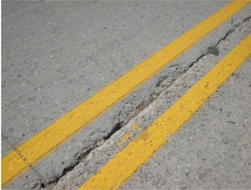
**Figure 65. Deteriorated Longitudinal Joint**
