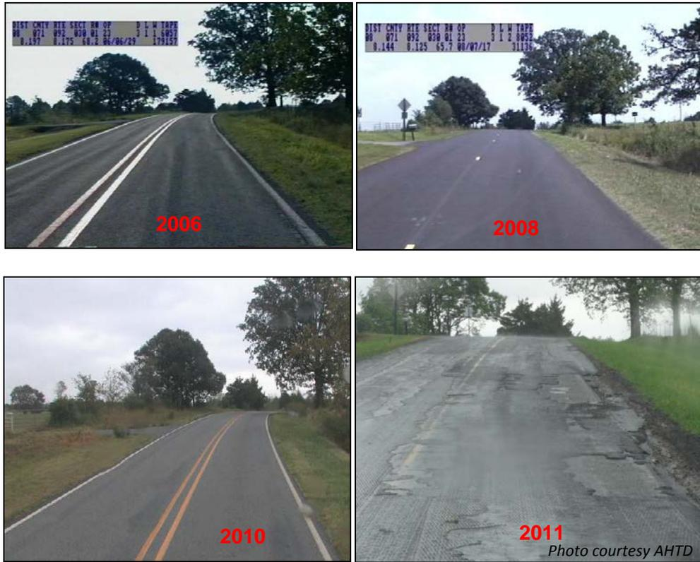
Figure 6. Typical Deterioration in the Fayetteville Shale Play Area (2006 - 2011)
