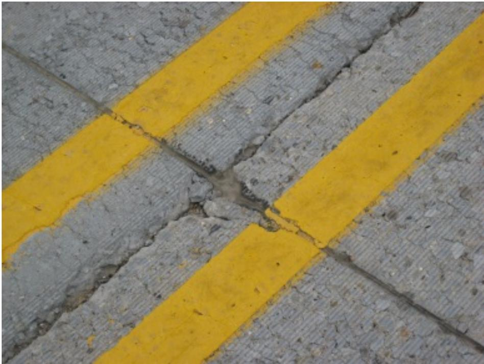
**Figure 64. Deteriorated Longitudinal Joint**
