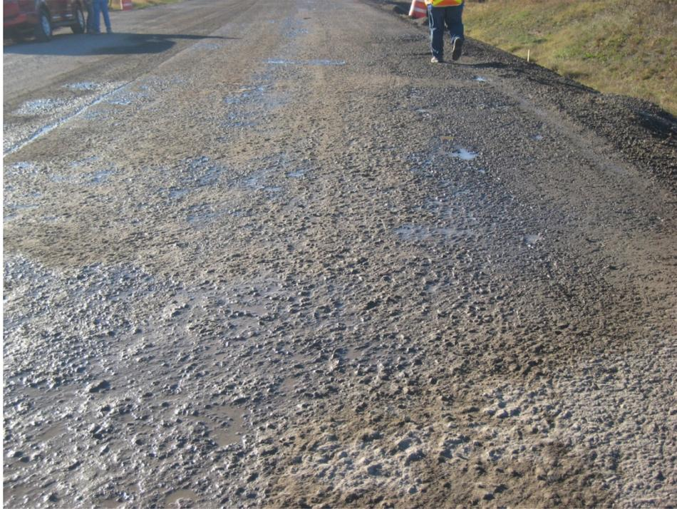
**Figure 23. CTRB Surface After Several Days of Traffic**
