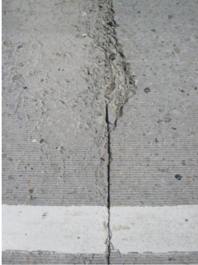
**Figure 56. Transverse Joint Deterioration**
