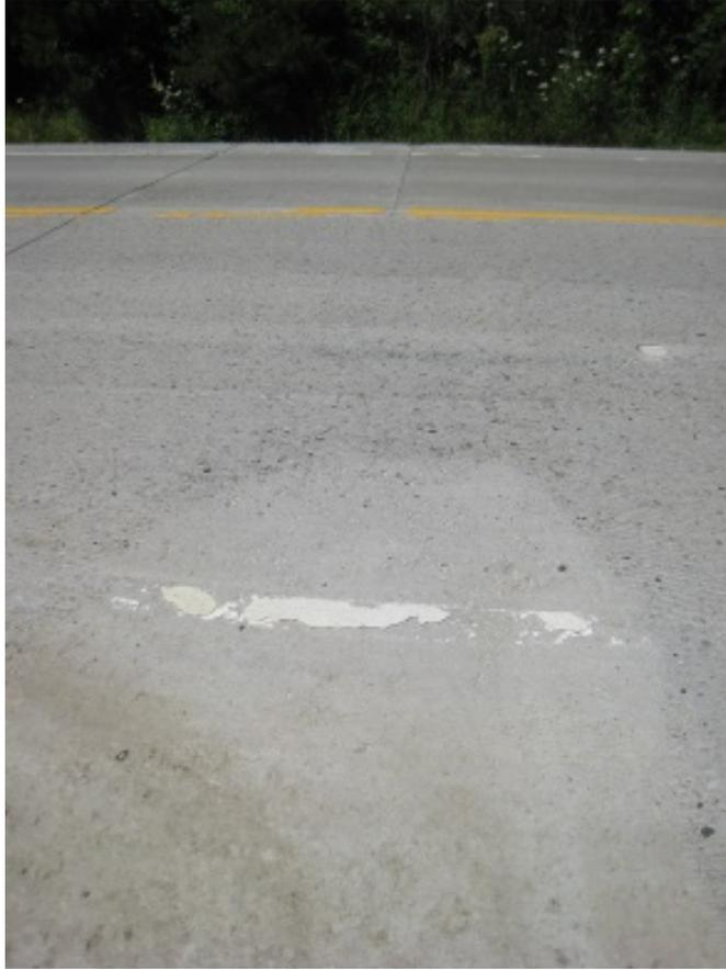
**Figure 88. Low Areas Remaining After Diamond Grinding**
