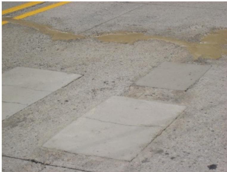
**Figure 54. Epoxy and Concrete Patches**
