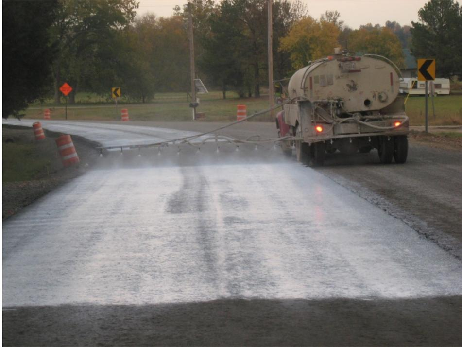
**Figure 29. Spraying Curing Compound on the Fresh RCC Mat**
