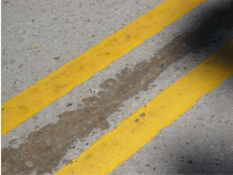
**Figure 60. Centerline Longitudinal Joint with Sealant**
