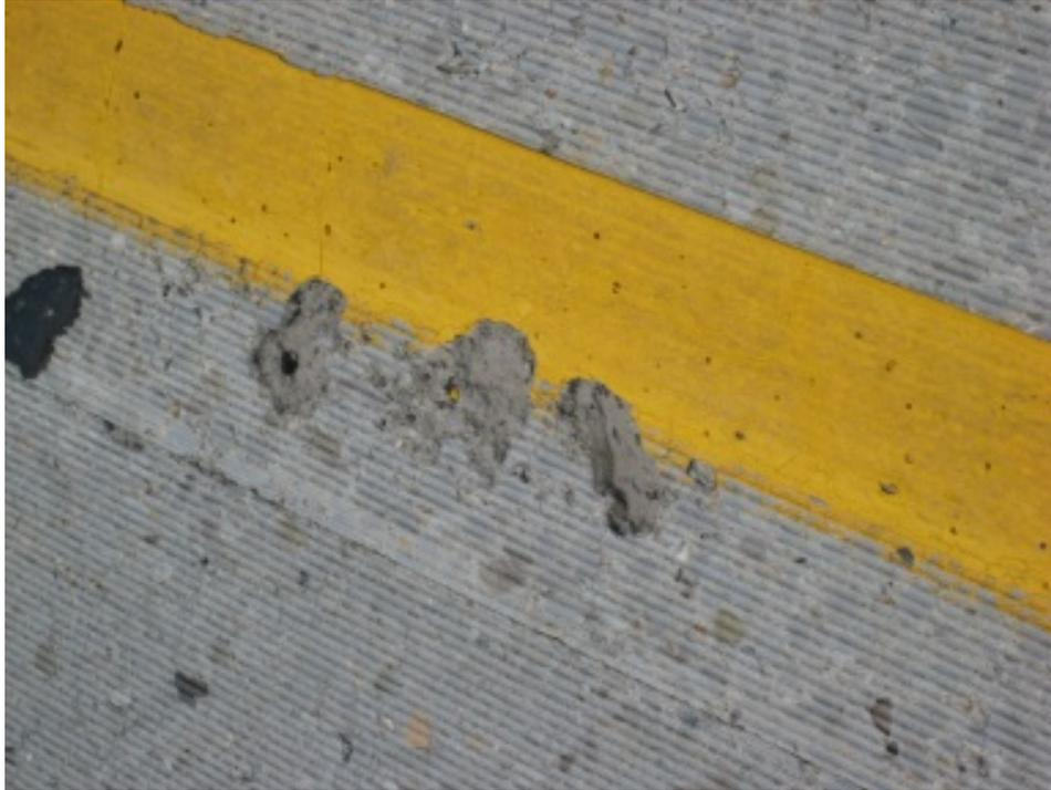
**Figure 78. Raveling in the RCC Surface**
