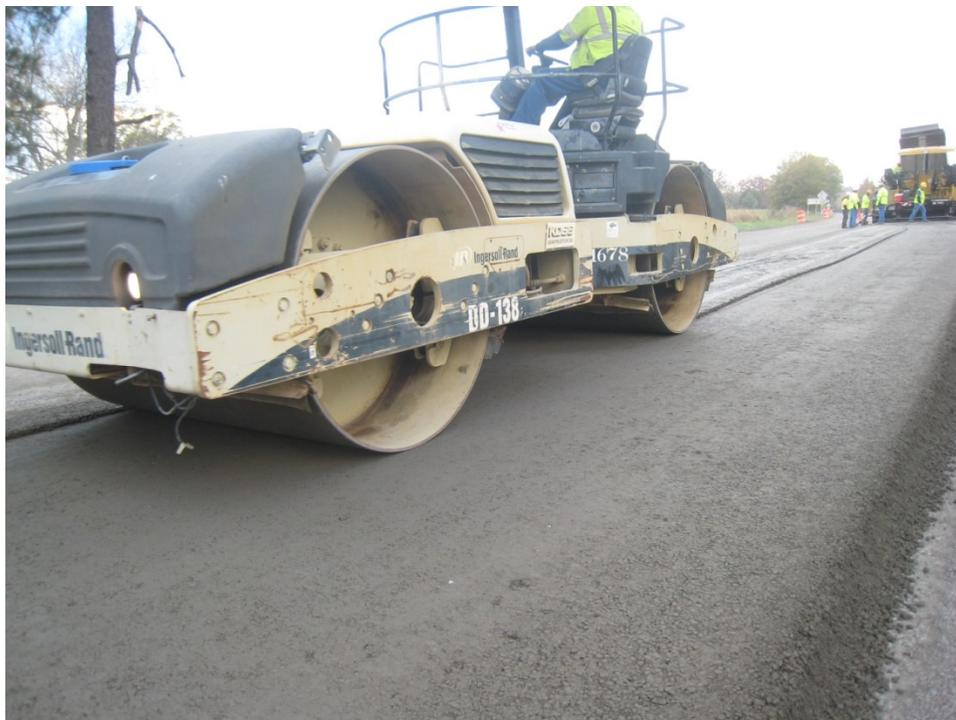
**Figure 28. Rolling the RCC Mat**
