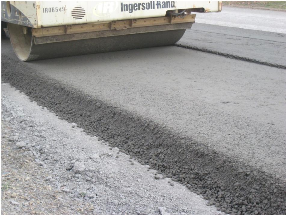
**Figure 27. Compacting the Edge of the RCC Mat with the Breakdown Roller**
