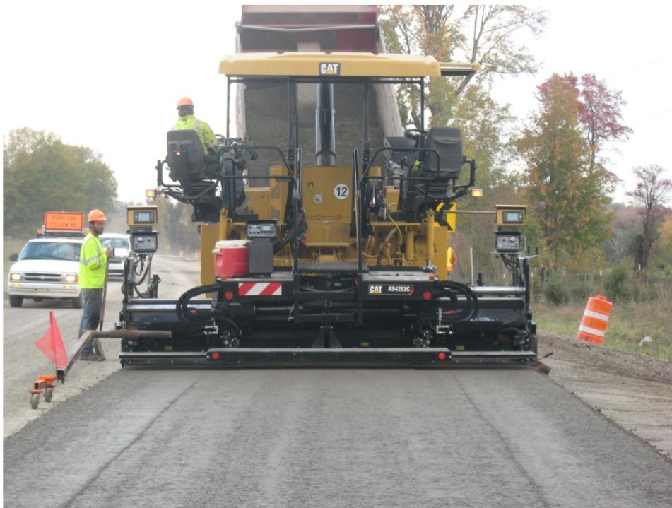
Figure 26. RCC Mat Behind the Paver
