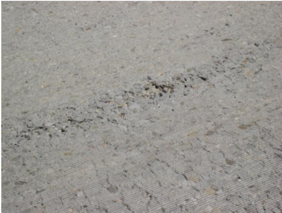
**Figure 77. Raveling in the RCC Surface**
