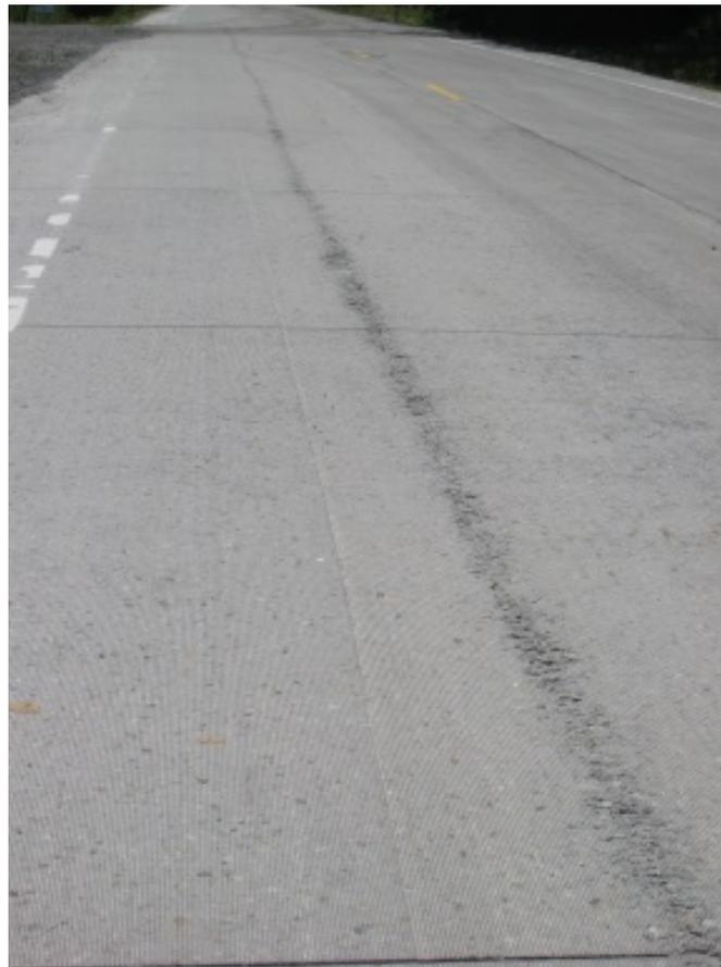
**Figure 82. Segregation in the RCC**
