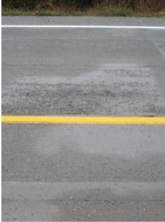
**Figure 79. Raveling in the RCC Surface**
