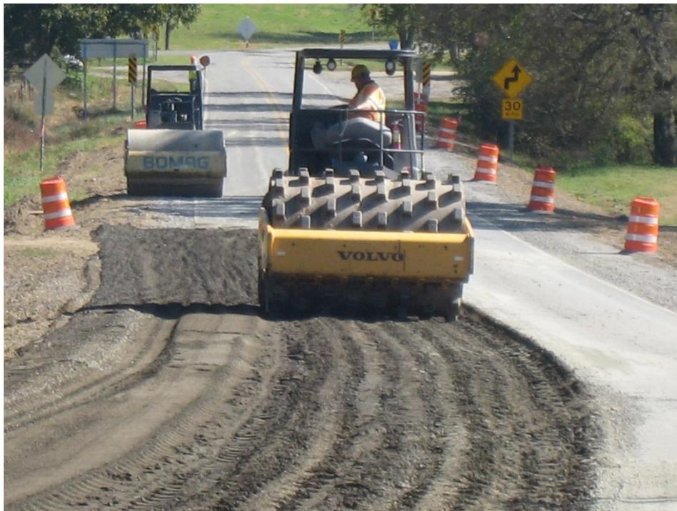
Figure 21. Compacting Mixed Base Material
