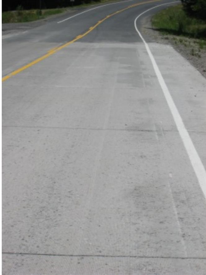
**Figure 87. Low Areas Remaining After Diamond Grinding**
