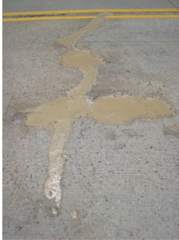
**Figure 53. Epoxy Patch at Construction Joint**
