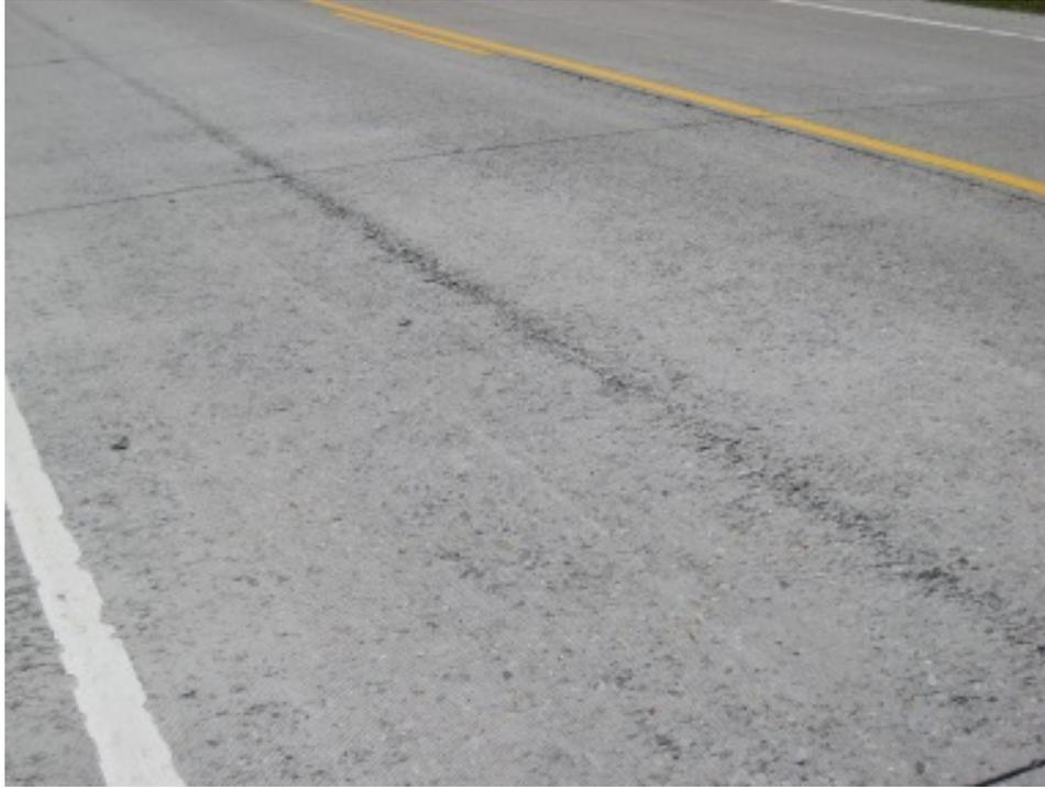
**Figure 83. Segregation in the RCC**
