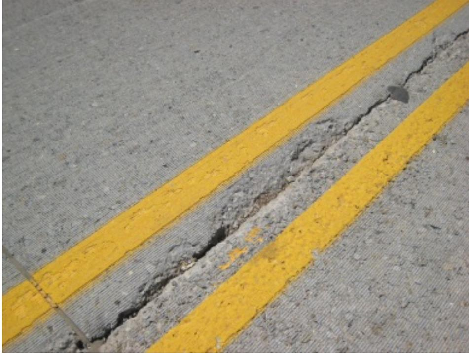
**Figure 65. Deteriorated Longitudinal Joint**
