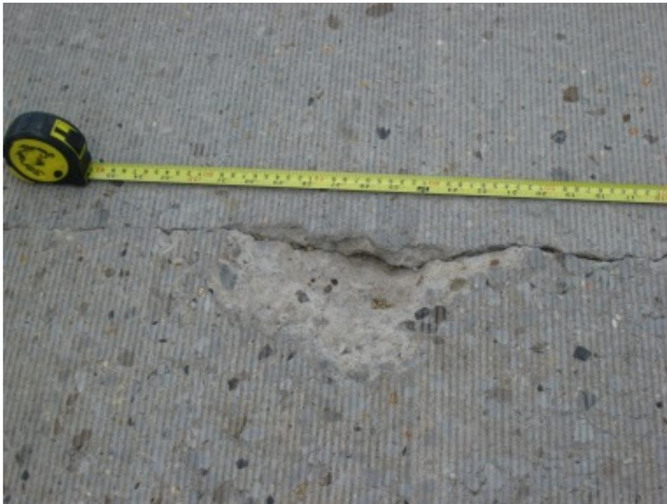
**Figure 58. Transverse Joint Deterioration**
