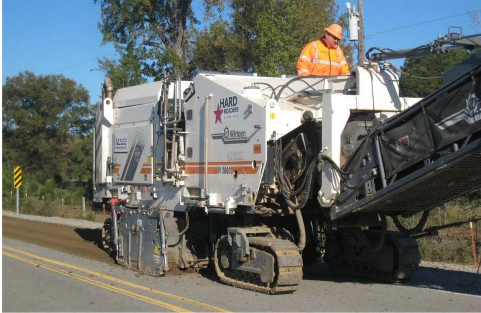
**Figure 18. Pulverizing Existing Asphalt Pavement**
