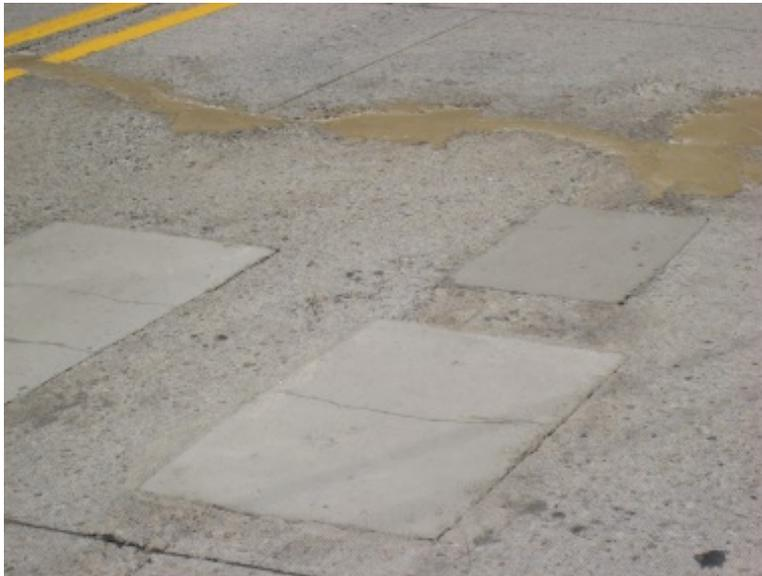
**Figure 54. Epoxy and Concrete Patches**
