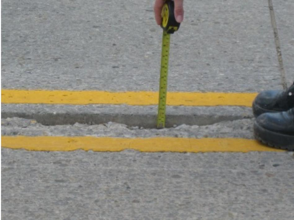
**Figure 63. Deteriorated Longitudinal Joint**
