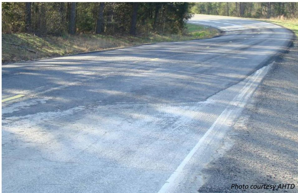
**Figure 3. Typical Roadway Distress in the Fayetteville Shale Play Area (Rutting with Patches)**
