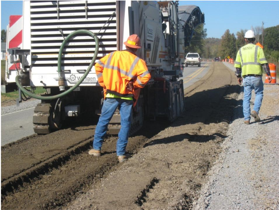
**Figure 17. Pulverizing Existing Asphalt Pavement**
