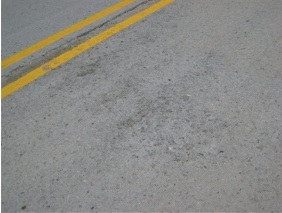
**Figure 76. Raveling in the RCC Surface**
