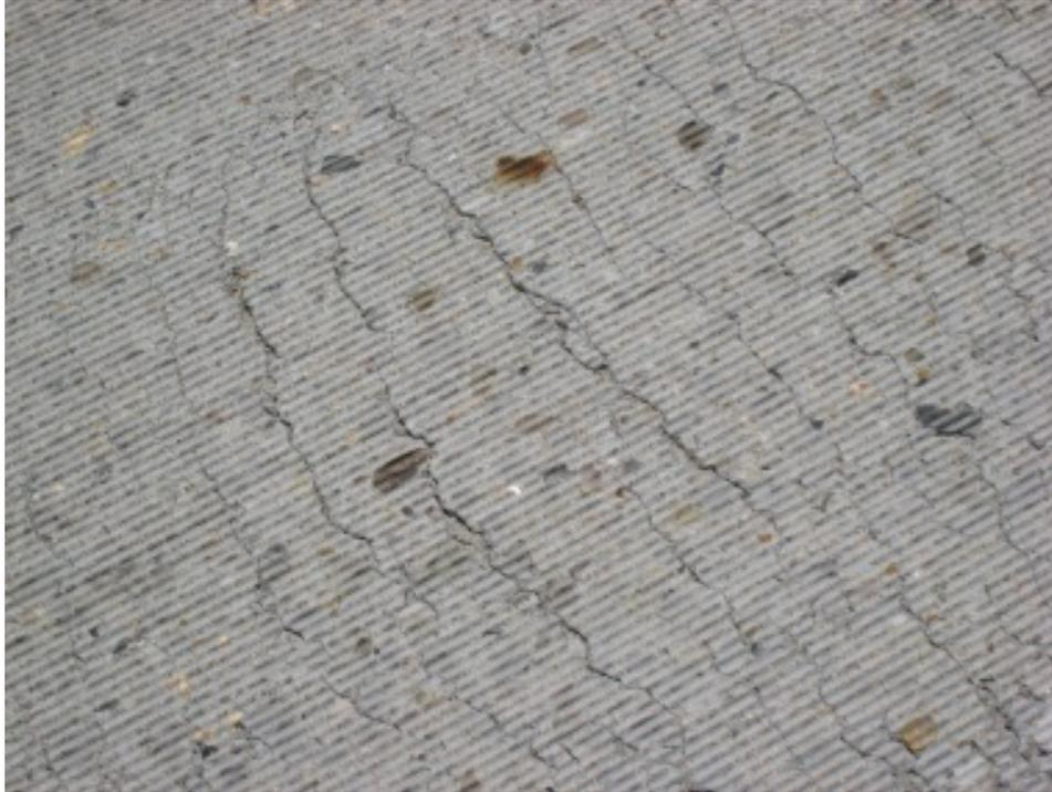
**Figure 86. Checking of the RCC Mat**
