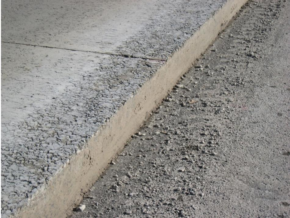
**Figure 33. Prepared Vertical Face at Longitudinal Joint**
