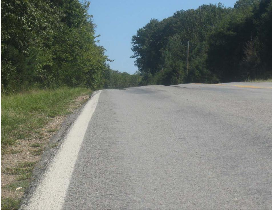
**Figure 8. Rutting on Highway 213**
