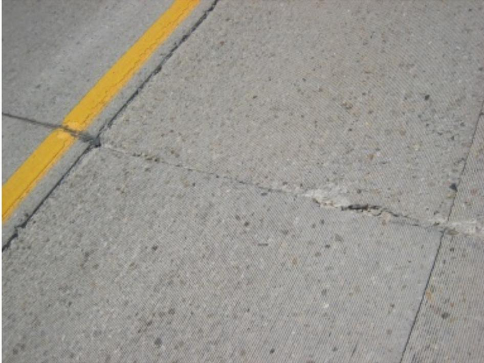
**Figure 57. Transverse Joint Deterioration**
