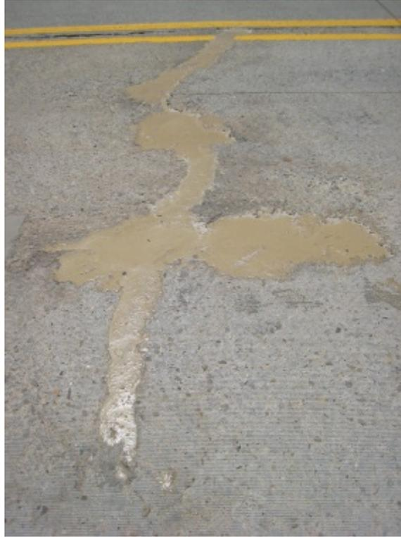
**Figure 53. Epoxy Patch at Construction Joint**
