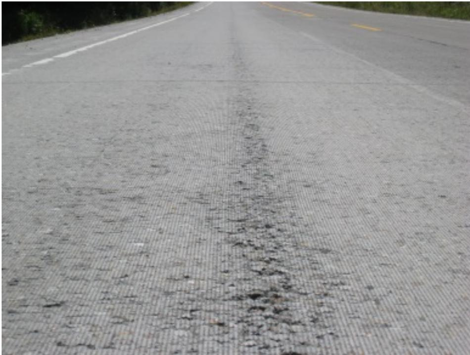
**Figure 84. Segregation in the RCC**
