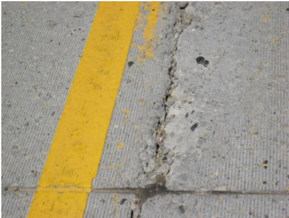
**Figure 62. Deteriorated Longitudinal Joint**
