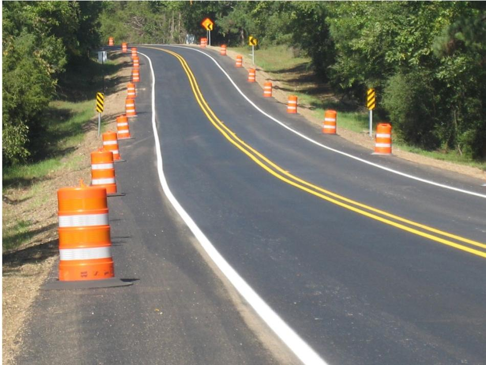
**Figure 39. Leveling Course Placed Prior to RCC Overlay**
