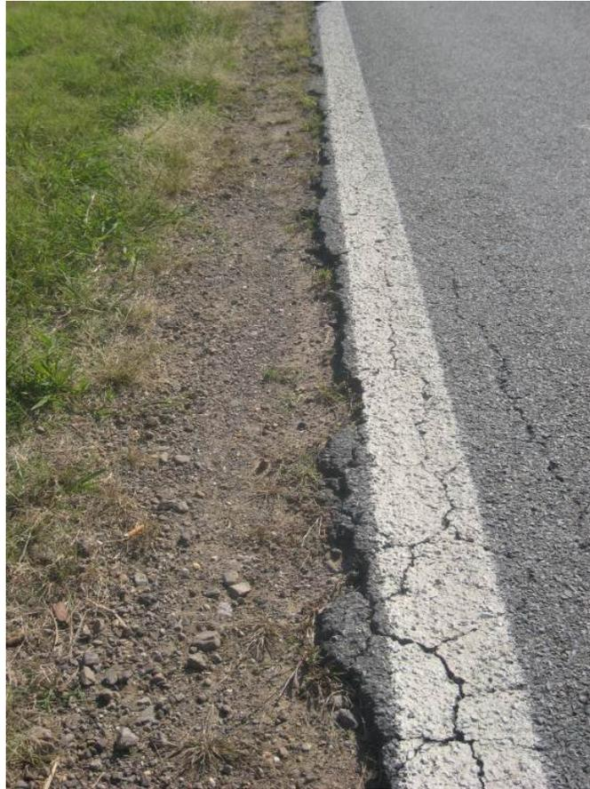
**Figure 9. Edge Cracking on Highway 213**
