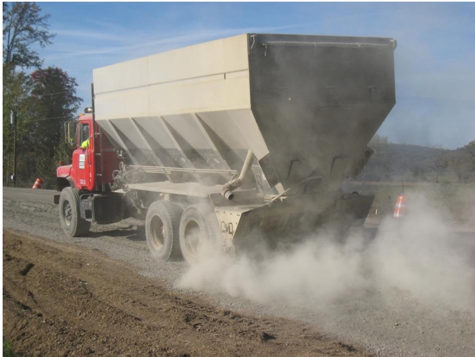
**Figure 19. Spreading Cement on Pulverized Material**
