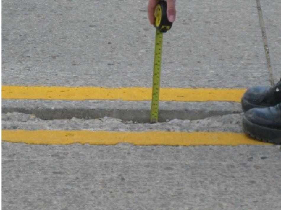
**Figure 63. Deteriorated Longitudinal Joint**
