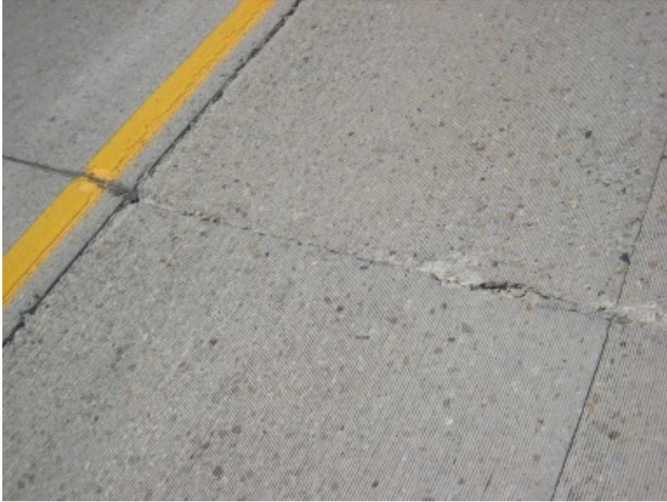
**Figure 57. Transverse Joint Deterioration**
