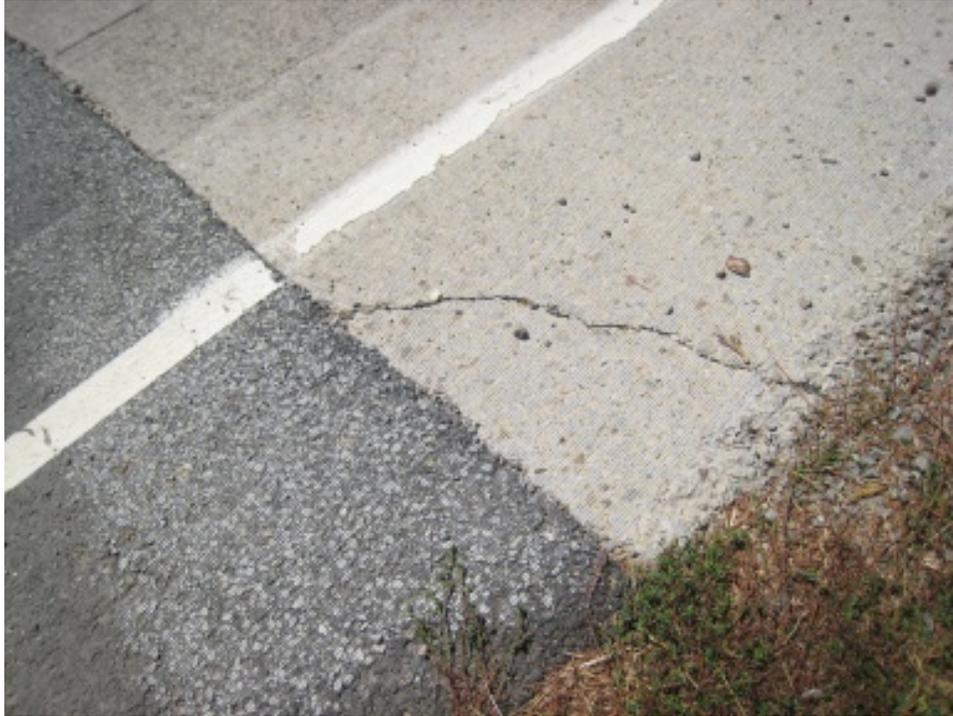
**Figure 67. Eighteen Inch Corner Crack – Sta. 187+00 WB**
