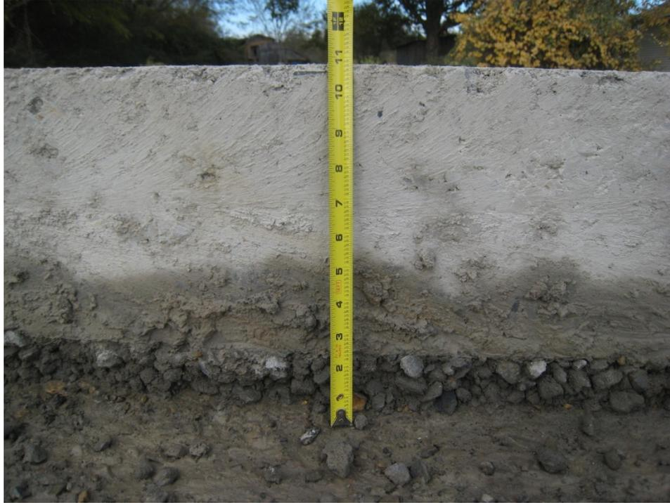
**Figure 31. Pavement Thickness of Approximately 11 Inches**
