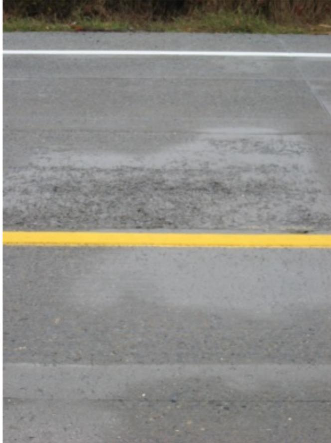
**Figure 79. Raveling in the RCC Surface**
