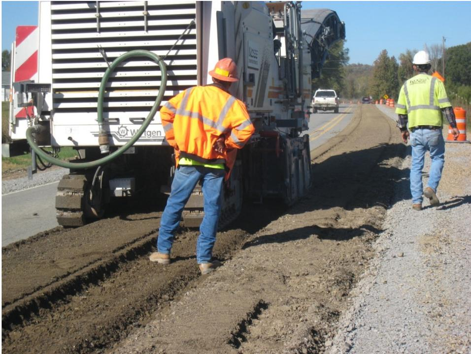
**Figure 17. Pulverizing Existing Asphalt Pavement**
