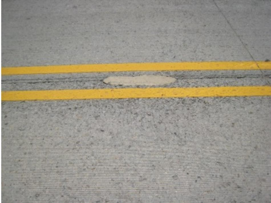
**Figure 61. Centerline Longitudinal Joint with Sealant**
