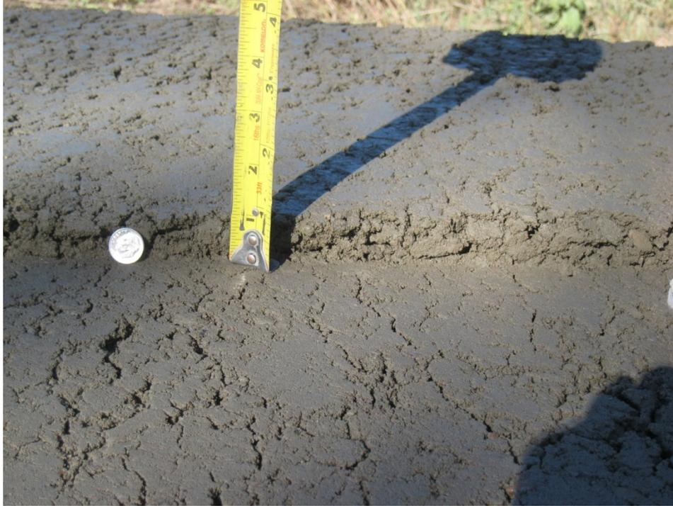
**Figure 30. Roll down of 1 Inch Achieved by Breakdown Roller**
