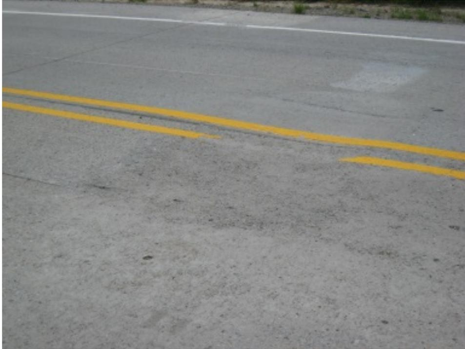
**Figure 89. Low Areas Remaining After Diamond Grinding**
