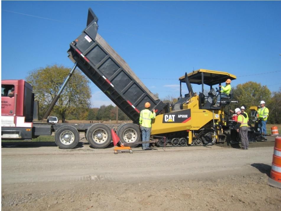
Figure 25. Loading the Paver Hopper Directly from the Truck
