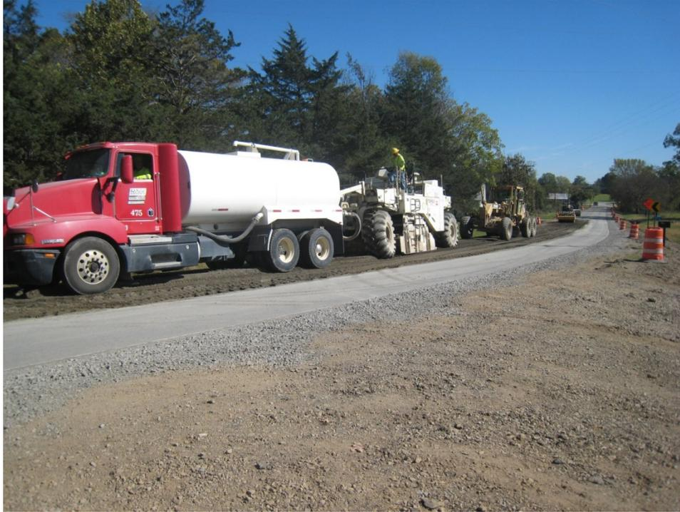
Figure 20. Mixing Pulverized Material with Cement and Water
