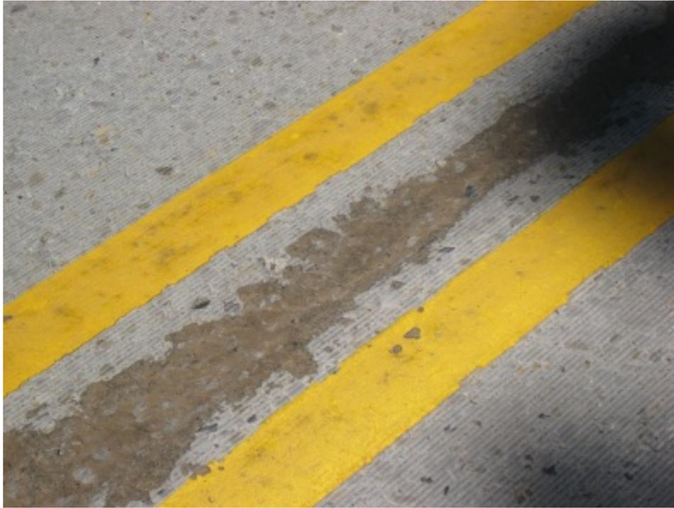
**Figure 60. Centerline Longitudinal Joint with Sealant**
