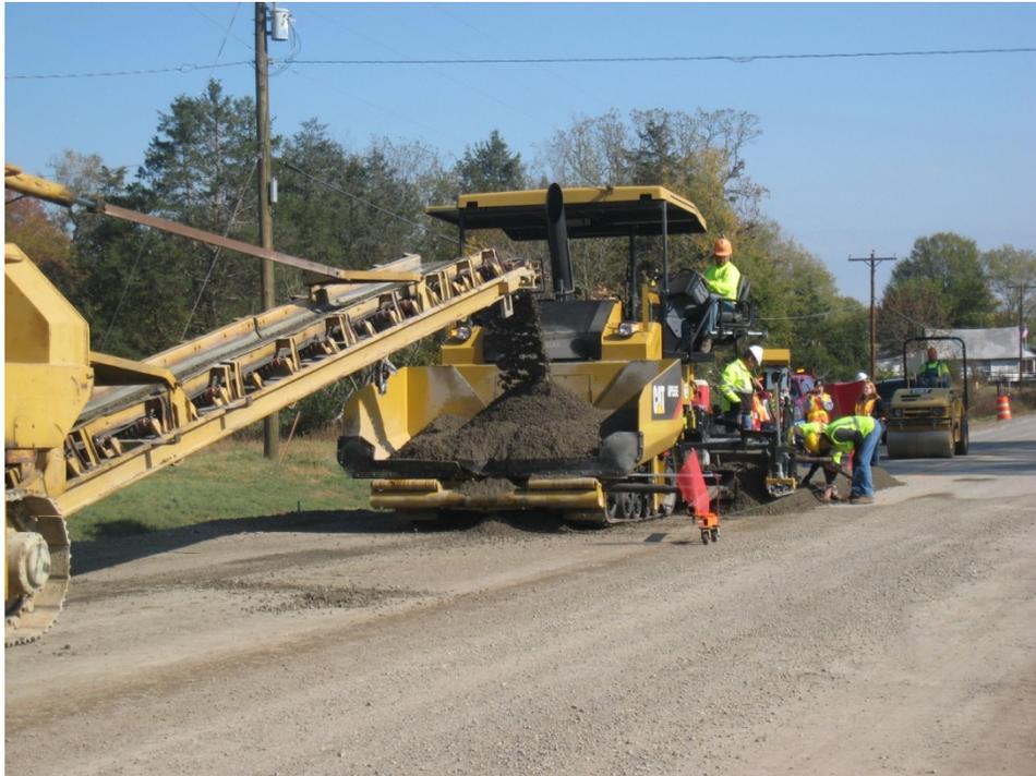
**Figure 24. Loading the Paver Hopper Using the Material Transfer Device**
