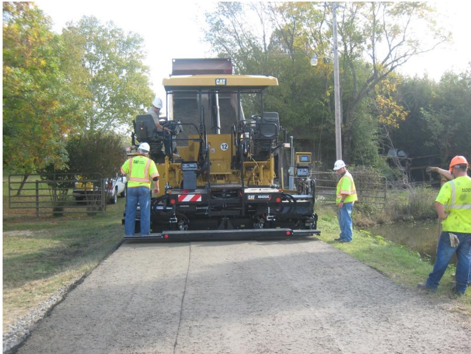
**Figure 16. Second Test Strip of RCC Placement (photo courtesy AHTD)**
