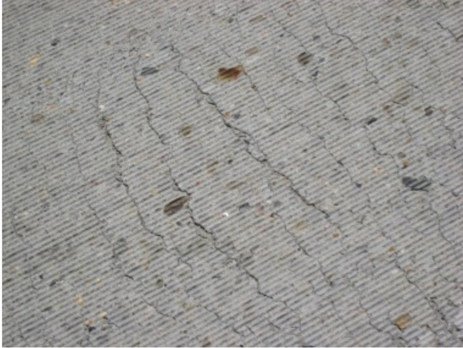
**Figure 86. Checking of the RCC Mat**
