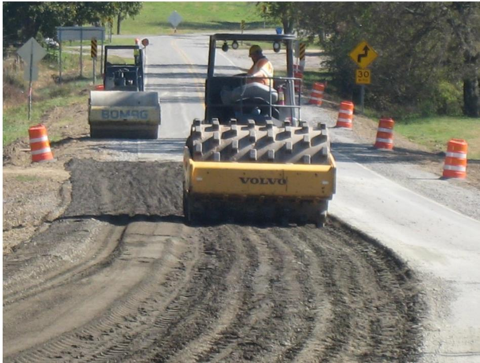
Figure 21. Compacting Mixed Base Material
