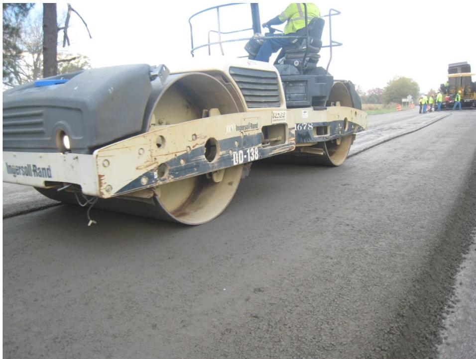
**Figure 28. Rolling the RCC Mat**
