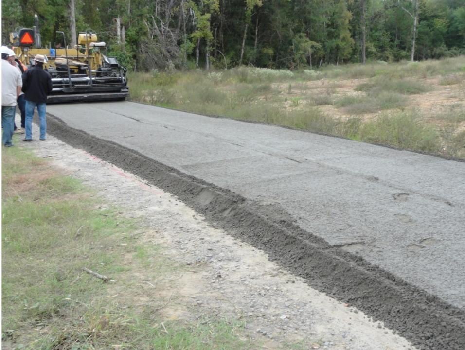
**Figure 15. First Test Strip of RCC Placement (photo courtesy AHTD)**
