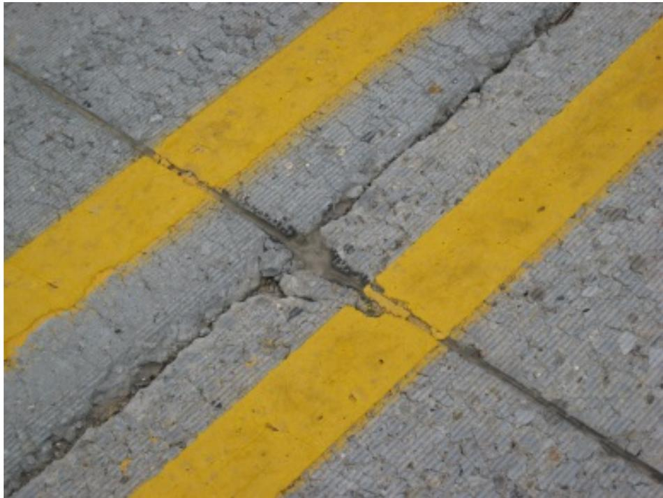
**Figure 64. Deteriorated Longitudinal Joint**
