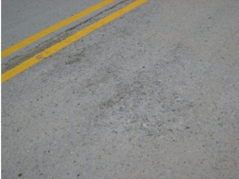
**Figure 76. Raveling in the RCC Surface**
