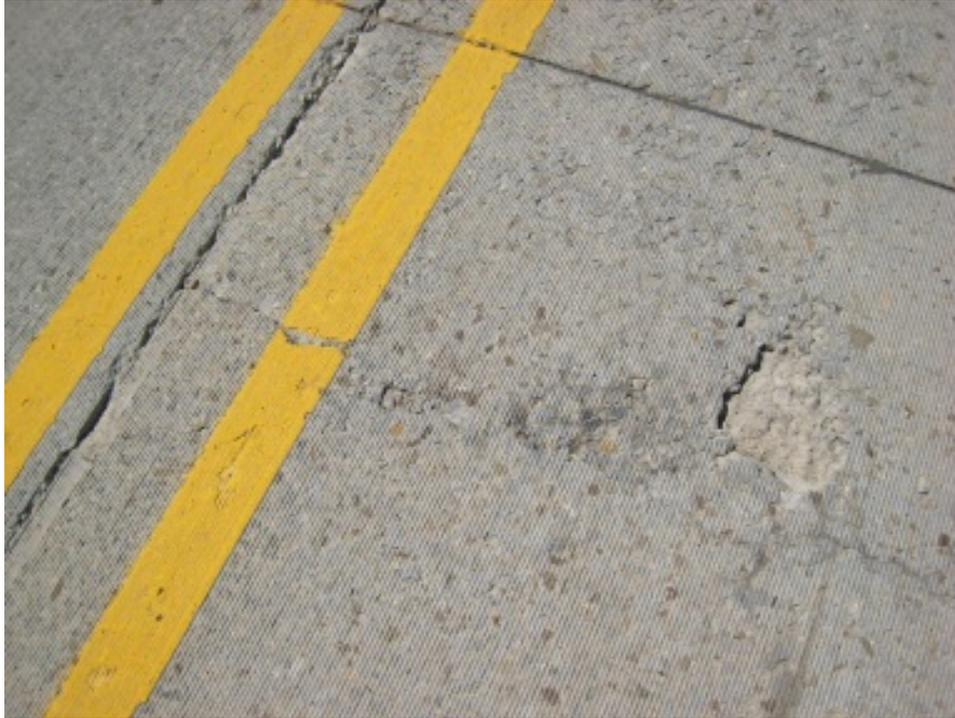
**Figure 69. 18-Inch Crack and Large Popout – Station 206+80**
