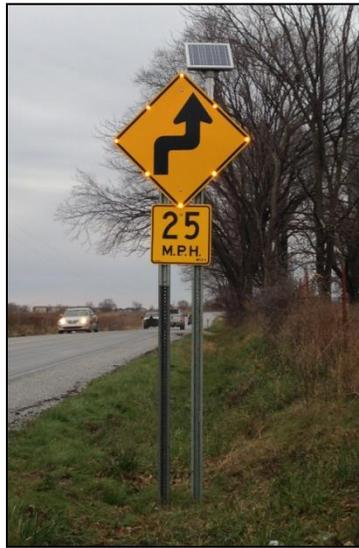
**Figure 7:** LED Curve Warning Blinker Sign
