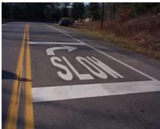
**Figure 1:** PennDOT Curve Advance Pavement Marking (Source: FHWA 2011)
