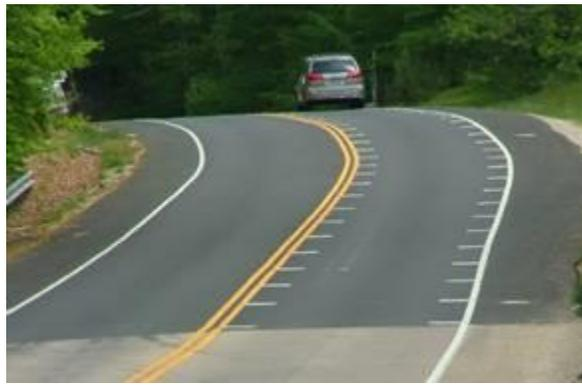
**Figure 4:** Optical Speed Bars Used to Reduce Vehicle Speed (Source: FHWA)
