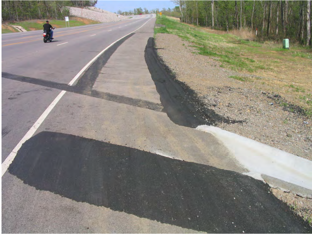
Figure 3.68 A site picture taken from the south to north.
