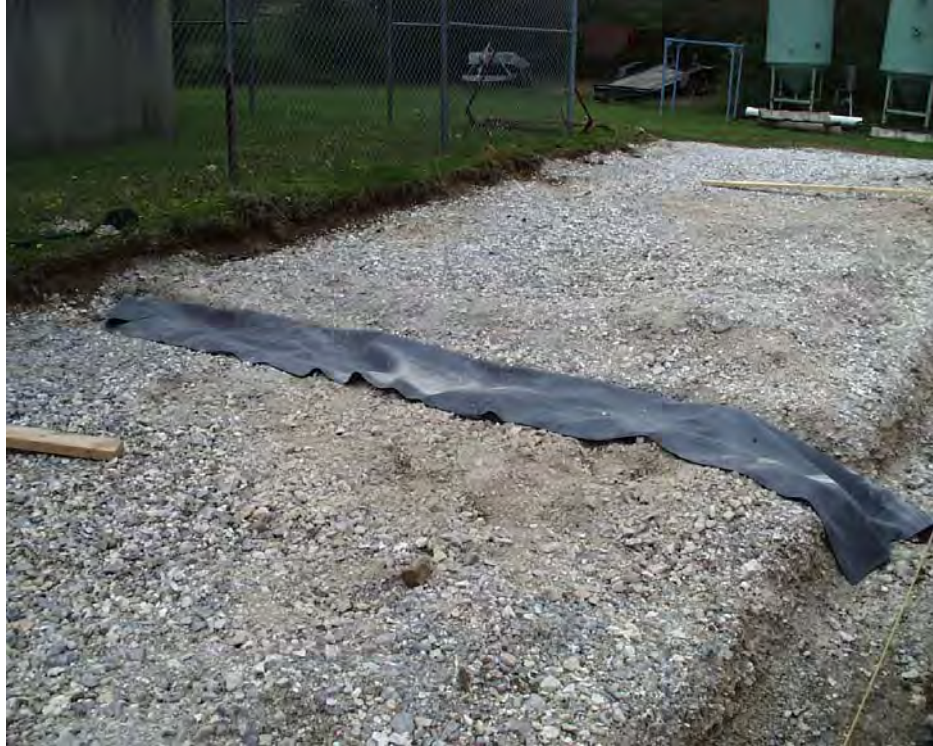
Figure 3.60 Surface of subbase course, a geomembrane separated the two test pads.
