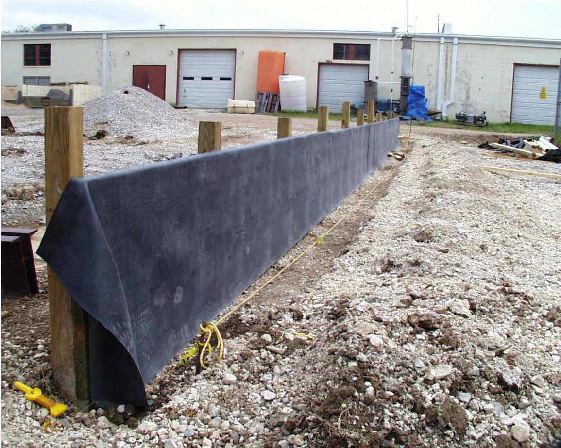
Figure 3.57 Waterproof retaining wall.
