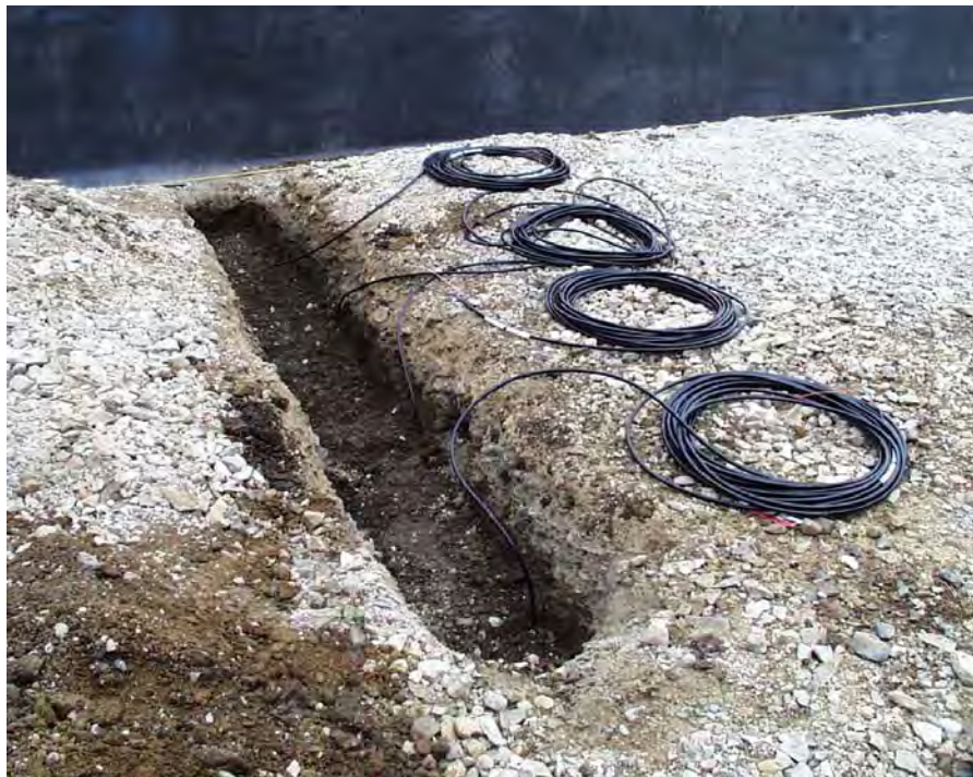
Figure 3.58 Installing moisture probes in subgrade soils.
