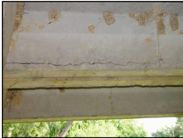
**Figure 5.14: Longitudinal Cracking on Danville PCB Bridge**
