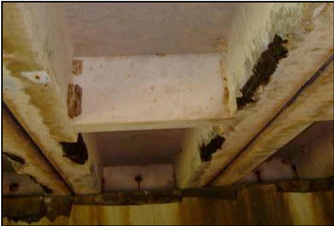
**Figure 10.4: Deteriorated Bridge Beam**
