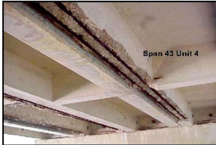
**Figure 4.1: Deterioration of Jenkins' Ferry Bridge**
