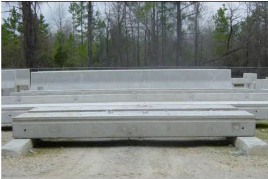
**Figure 2.10: Newly Fabricated Precast Channel Beam**
