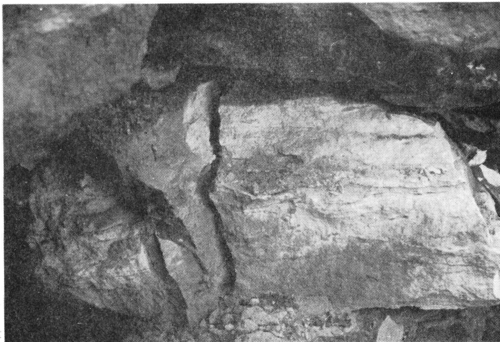
Figure 2.2 Cracked Stone in the Wall.
