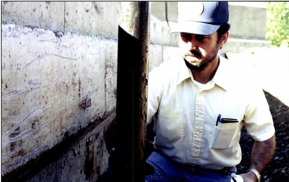
Figure 10. The grease used to keep the steel risers from sticking to the surrounding medium can be seen.
