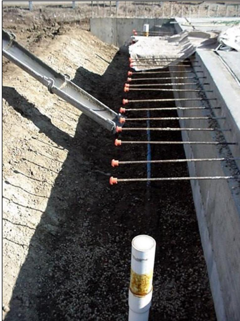
**Figure 22. Final placement of the horizontal inclinometer tube and settlement plates at the southern embankment of the Crow Creek Bridge.**
