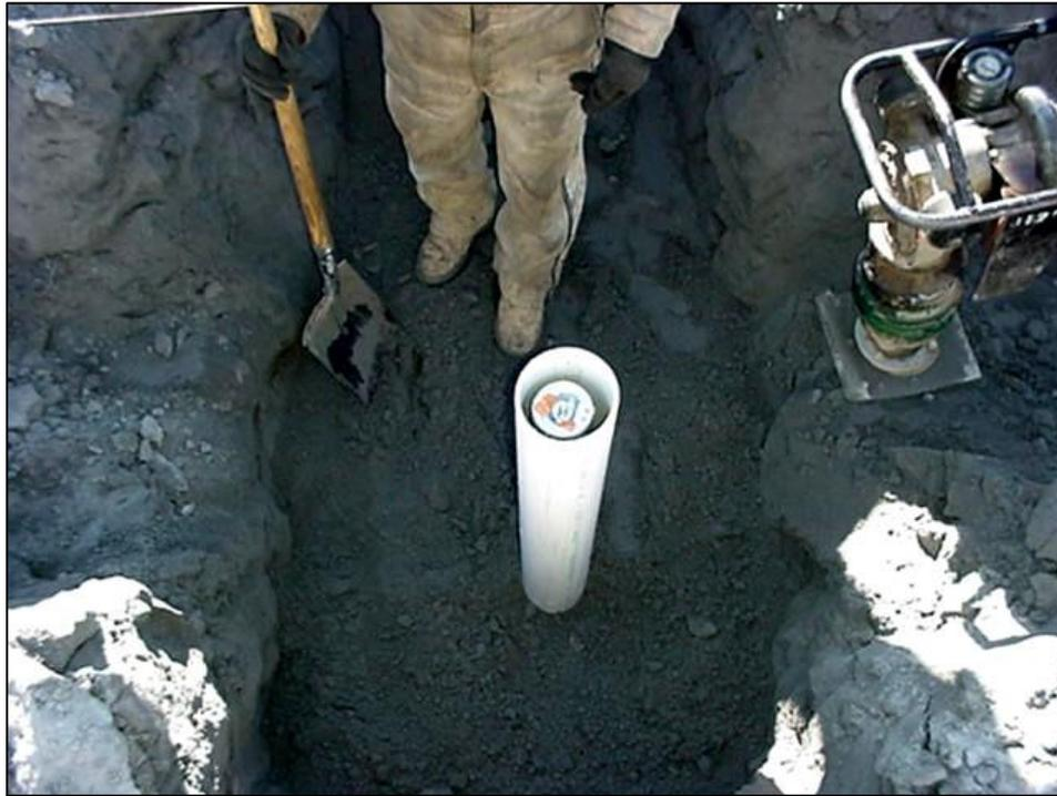
**Figure 16. PVC riser in the compacted fill embankment at Chicot Road.**
