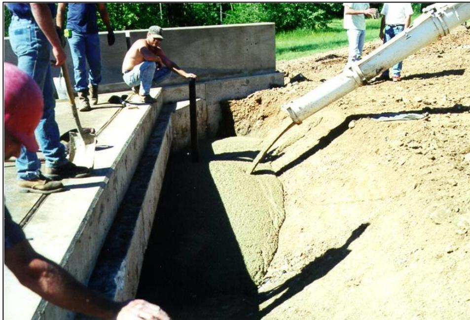
Figure 8. Flowable fill filling the embankment trench at the west embankment of the DeRoche Bayou Bridge.
