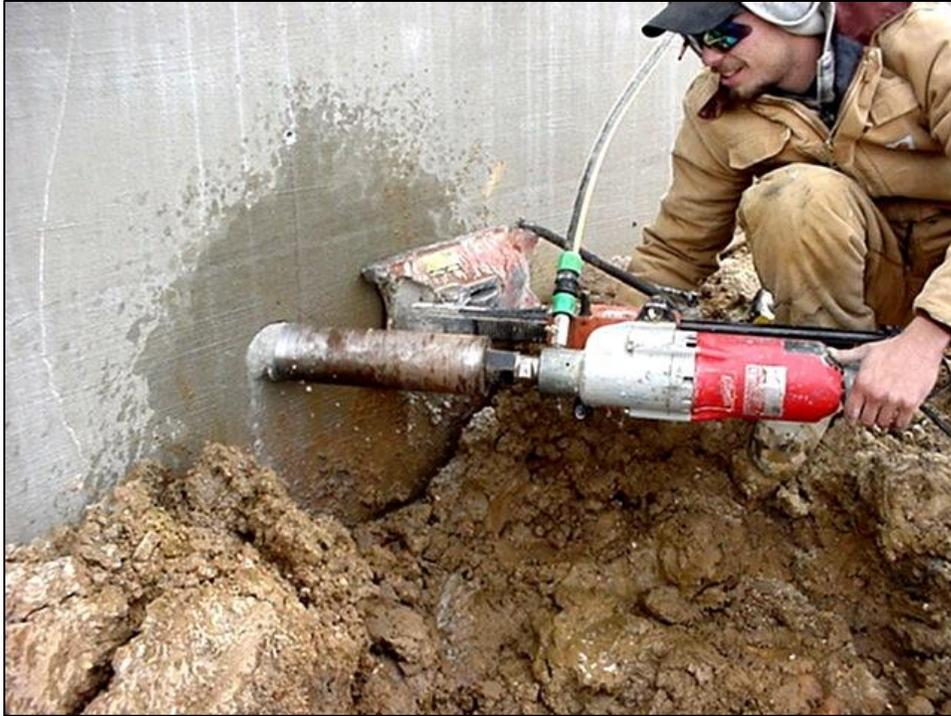
Figure 17. Drilling through a wingwall for horizontal inclinometer installation.
