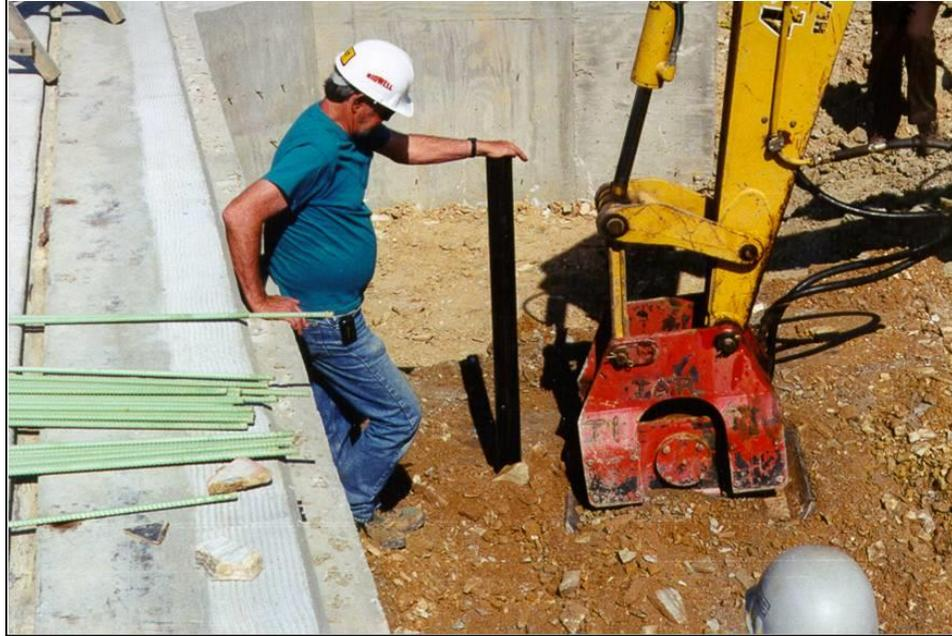
**Figure 12. Compacting the earth around a steel riser at Raymar Road.**
