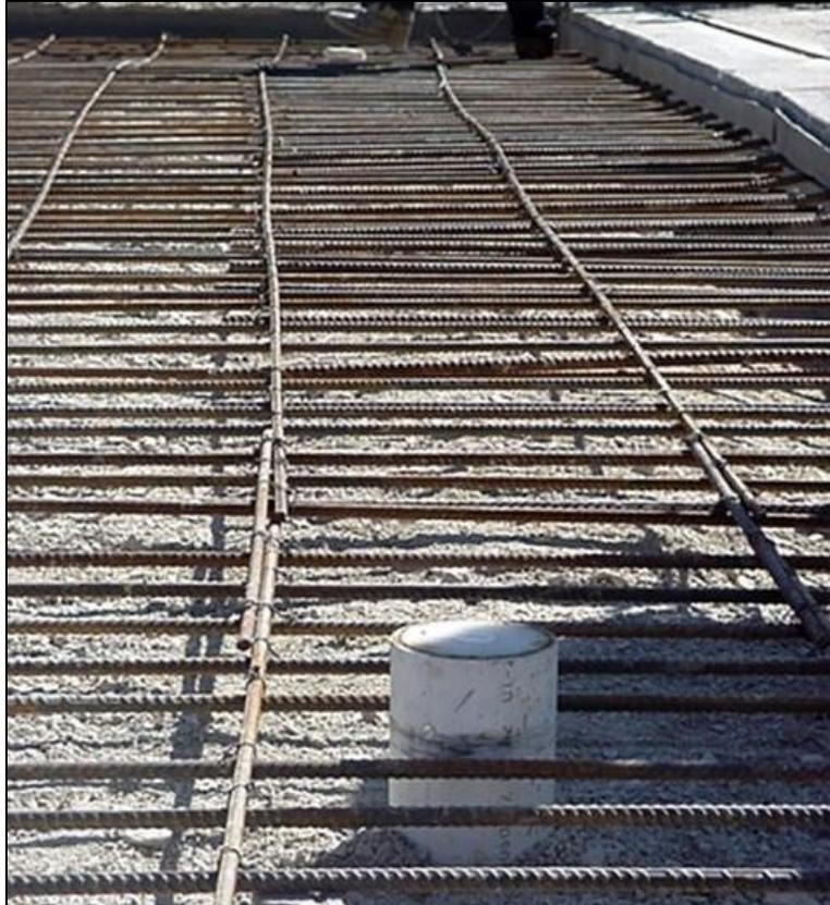
Figure 24. Capped access tubes sticking up between reinforcing members.
