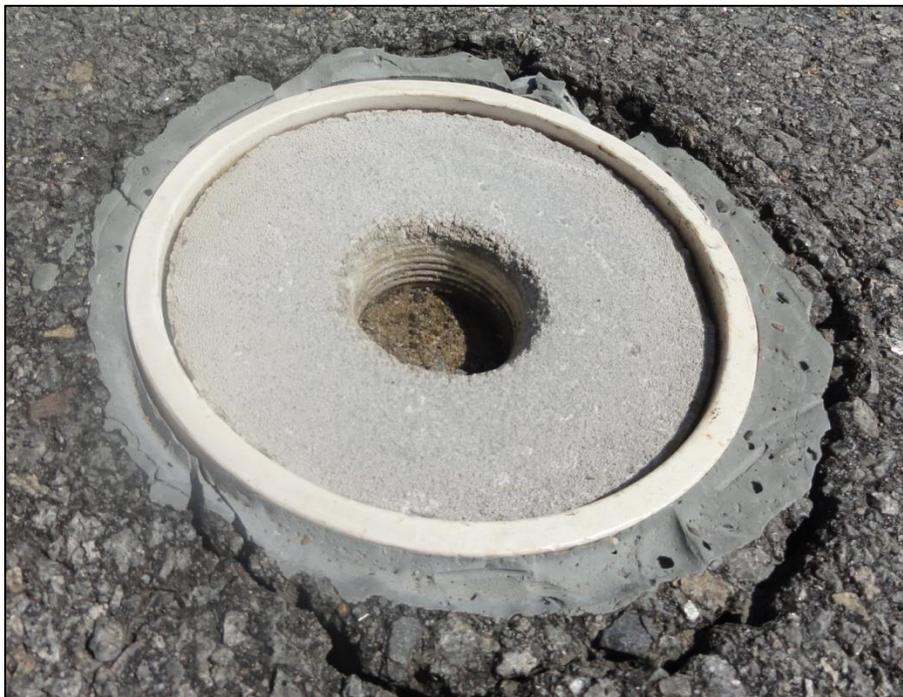
Figure 26. Dilapidated cap after ten years of neglect.
