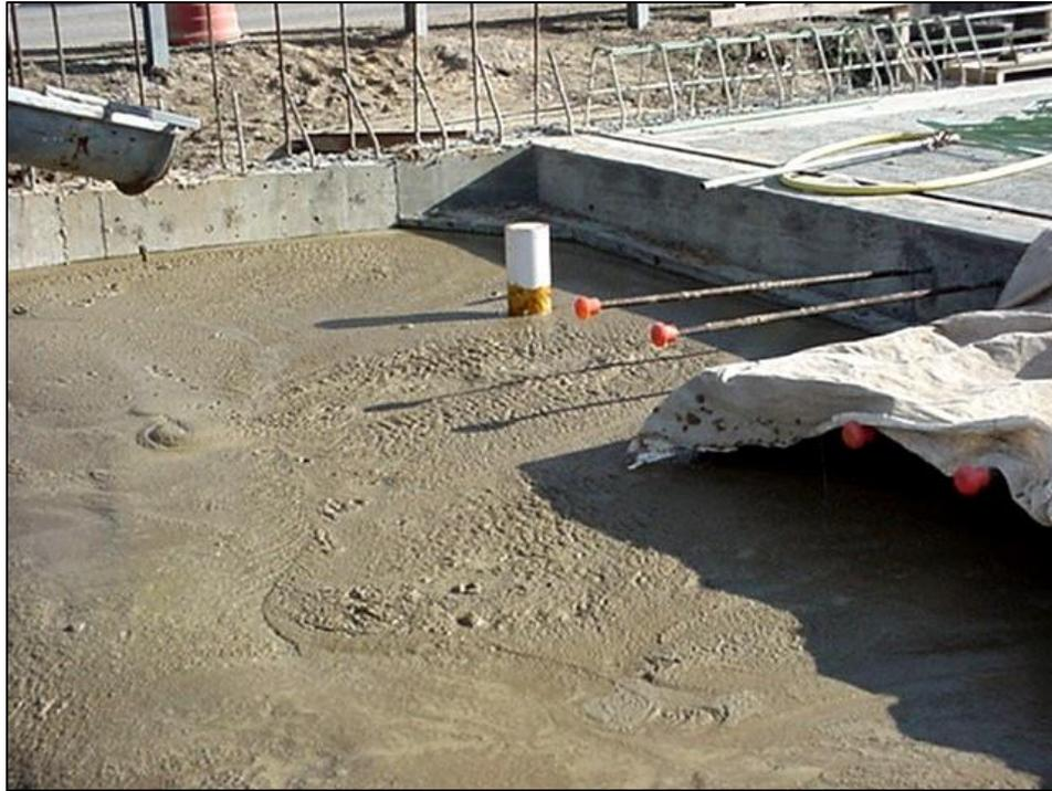
**Figure 23. Flowable fill poured at the southern embankment of the Crow Creek Bridge.**
