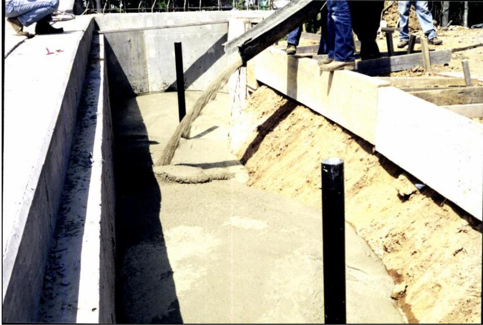
**Figure 13. Flowable fill being added to the north embankment of the Raymar Road Bridge.**
