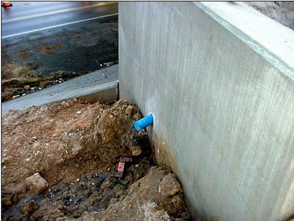
Figure 18. Horizontal inclinometer tube protruding from a wingwall.
