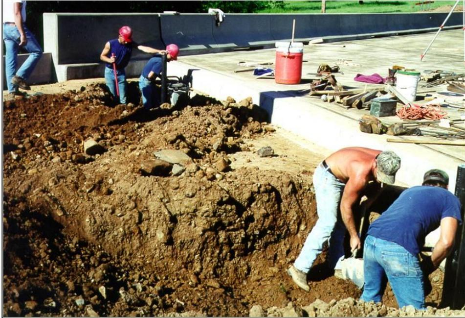
Figure 9. Compacted fill at east embankment of the DeRoche Bayou Bridge.
