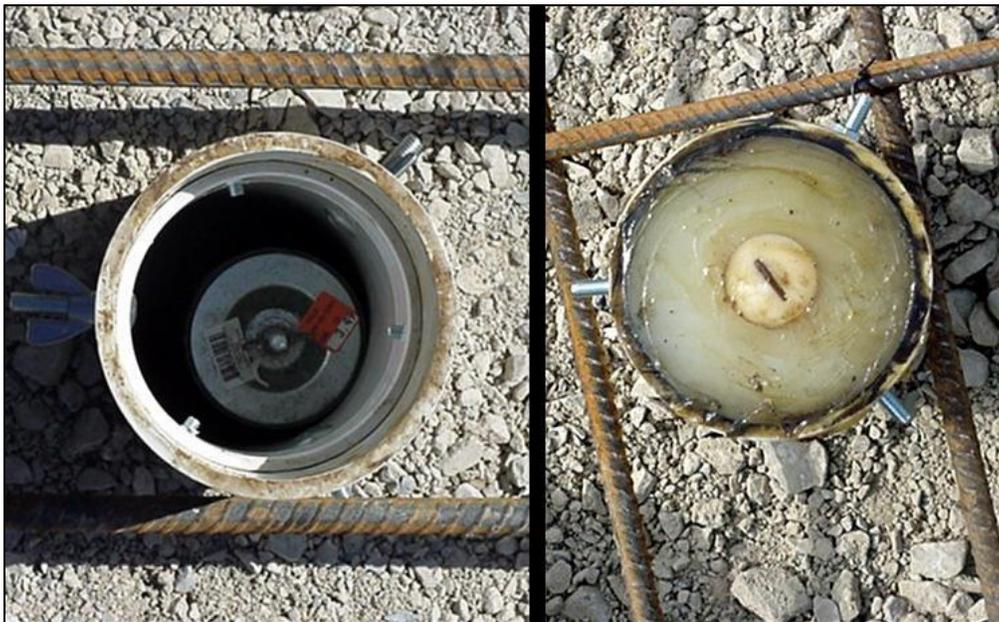
Figure 25. PVC riser in the access tube (left) and a greasy polypropylene cap (right).
