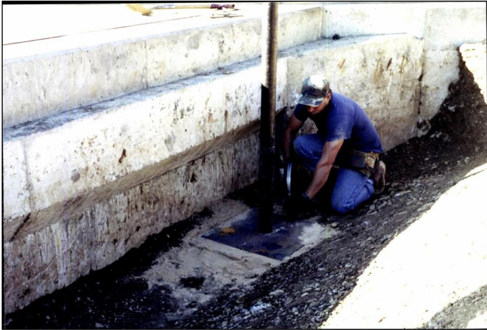
Figure 7. The settlement plates were bedded on sand and staked with rebar.
