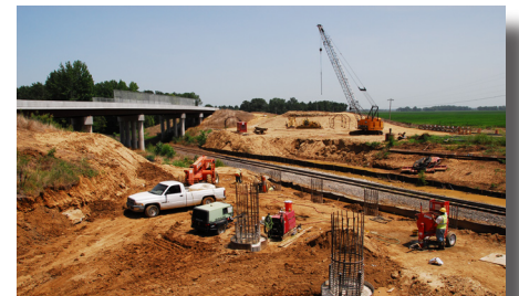
Widening of Highway 1 near Marianna.
