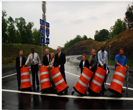
The new Interstate 40 Interchange at Conway.
