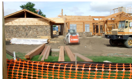
Construction of the new Arkansas Welcome Center at Blytheville.
