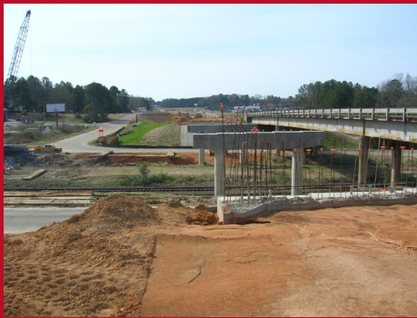
Widening on Highway 167 in El Dorado.
