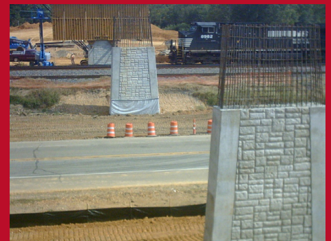
Highway 67 overpass in Prescott.
