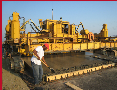
Widening on Highway 65 in Lincoln County.
