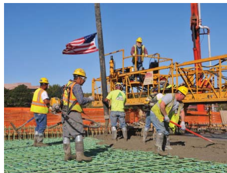
Interstate 430/630 interchange, Little Rock
