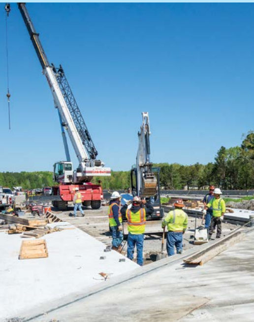
Rehabilitating Interstate 530 in Jefferson County
