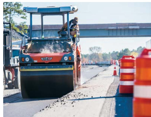
Widening of Interstate 40 in Pulaski County
