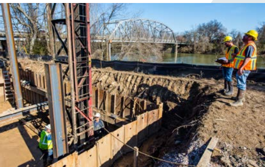
Highway 51 Ouachita River Bridge
