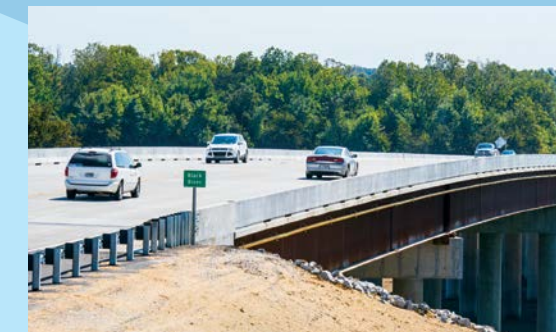
Highway 63 Bridge at Black Rock
