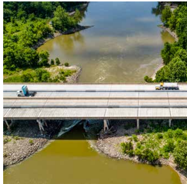
Interstate 555 in Poinsett County
