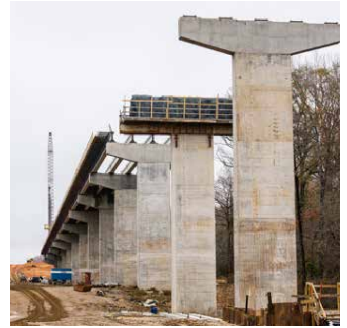
State Highway 51 Bridge across Ouachita River at Calion
