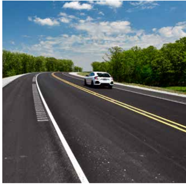
State Highway 13 – Searcy Bypass
