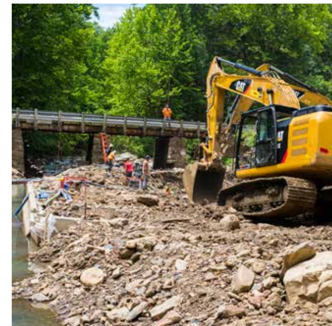
State Highway 123 in Johnson County
