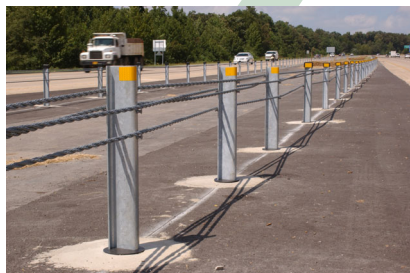
The new safety fence on Interstate 430 in Little Rock.
