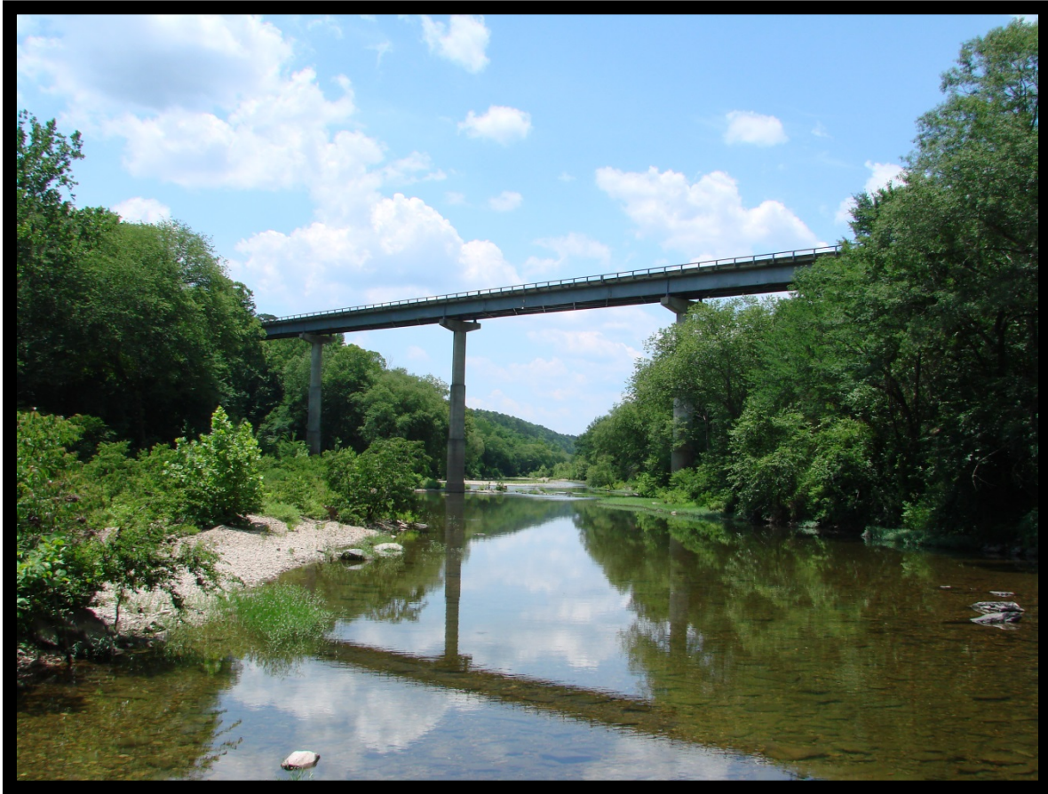
Figure 1: Cossatot River Bridge (ARDOT Bridge Number 05686)
