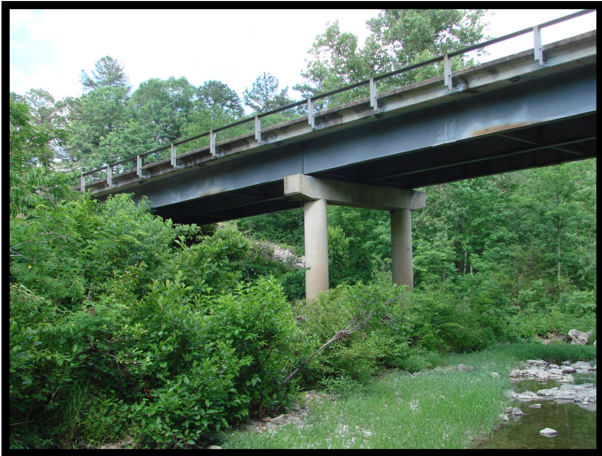
Figure 2: Baker Creek Bridge (ARDOT Bridge Number 05687)
