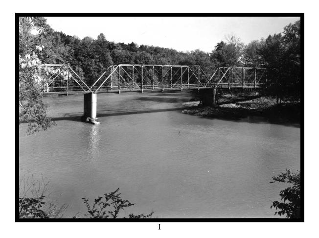
ARDOT Bridge Number 13091, on Wire Road, was listed in the National Register of Historic Places in 2007. The Lakeside Bridge and Steel Company of Milwaukee, Wisconsin, erected two spans of this bridge over the Mulberry River in 1929. The Great Flood of 1927 damaged the previous bridge (built circa 1912); one span of that 1912 structure might be the westerly span of the present bridge. The bridge was rehabilitated in 1976 and had extensive repairs in 2006.
