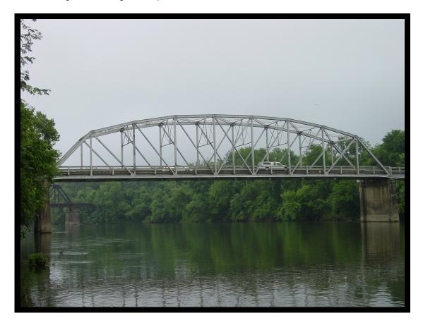
The Ouachita River Bridge (ARDOT Bridge Number 01412) is located in Clark County over the Ouachita River, previously carrying Highway 51. The Luten Bridge Company of Little Rock, Arkansas built the steel, Parker through truss bridge in 1933 over the Caddo River. The truss span was moved to its current location in 1960, which illustrates the versatility and portability of truss bridges.
