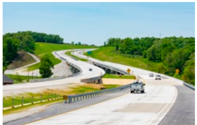
LOCATION: Springdale, AR • CONTRACTOR: Eutaw Construction COST: $104.3 million • LENGTH: 4.5 miles • COMPLETION DATE: 4/29/18
